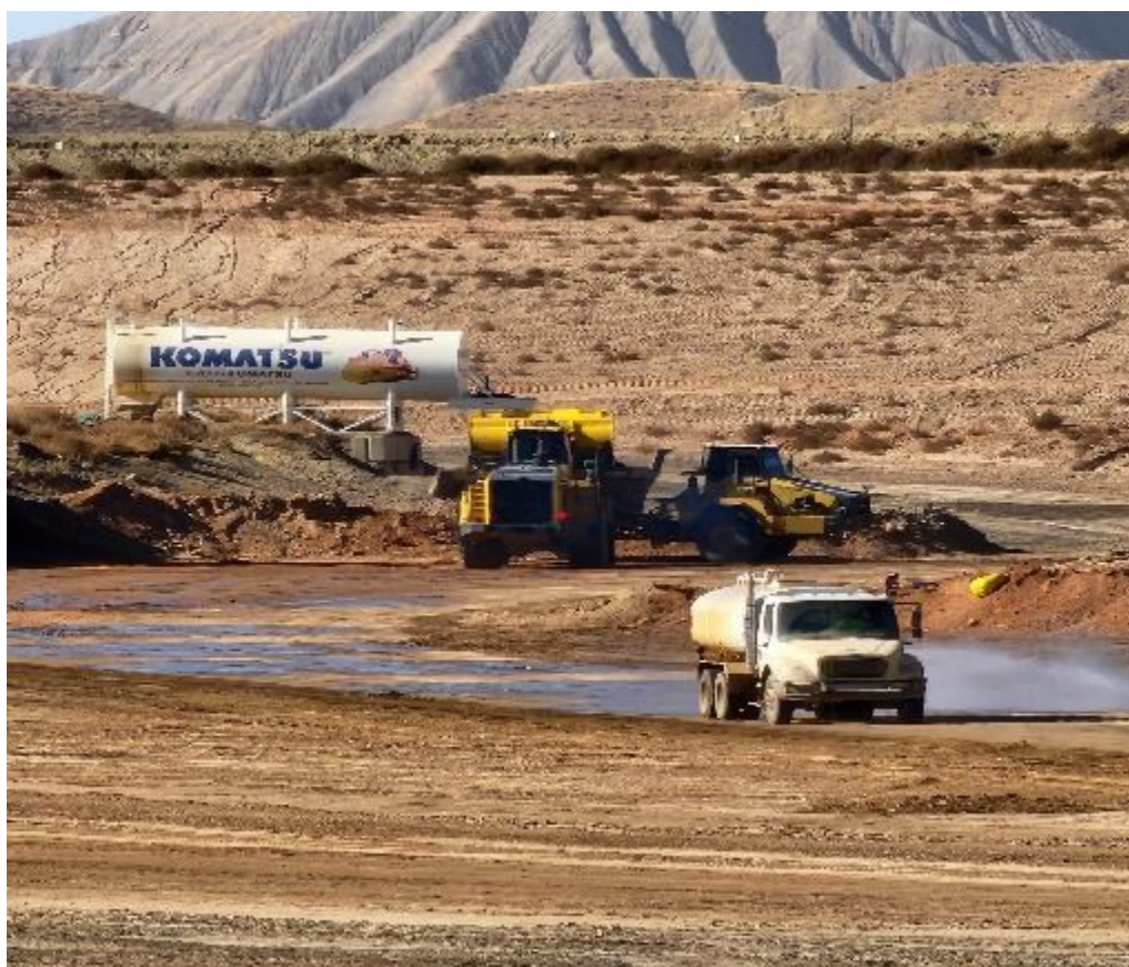
Photo 4. Dust control in cell November 2023
