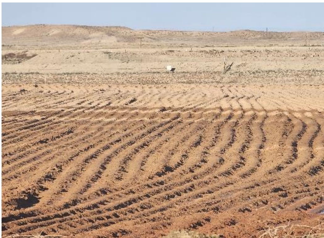
Photo 25. Scarified TOW prepped for Interim Cover placement July 2024
