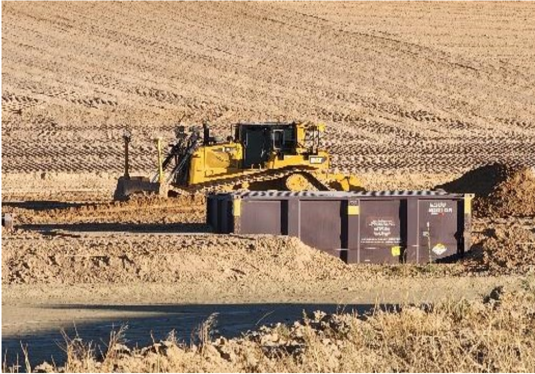
Photo 19. Placing RRM around containers July 2024
