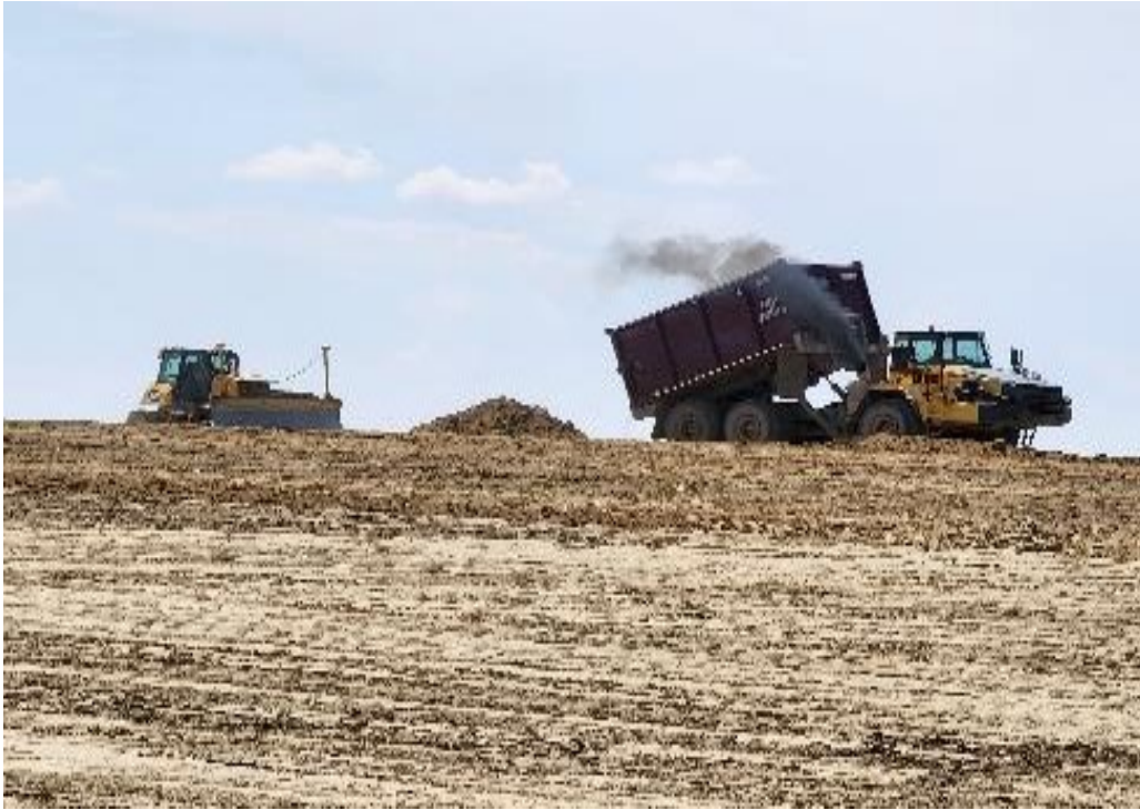
Photo 31. Placing protective cover on Interim Cover August 2024
