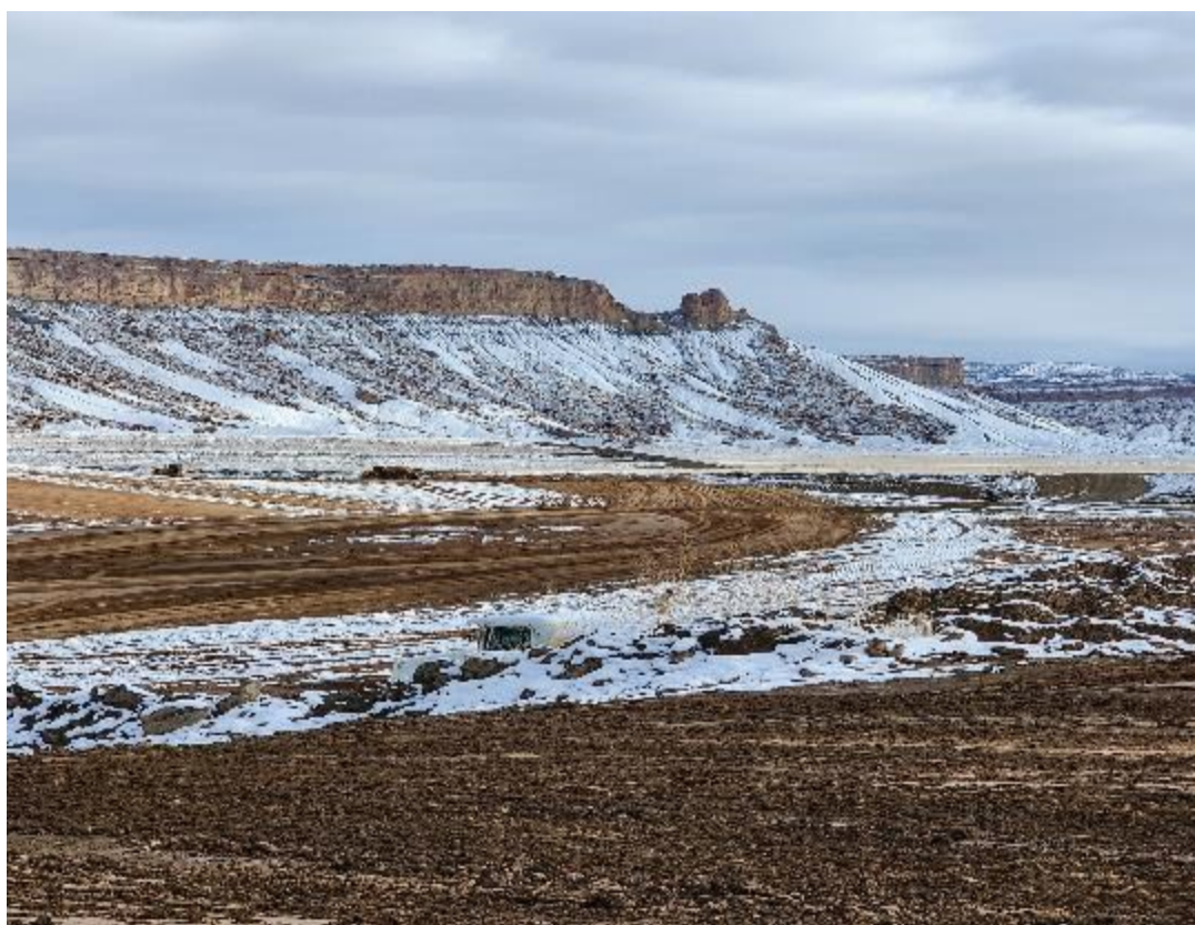
Photo 12. Dozer cleaning snow off lifts before placement March 2024
