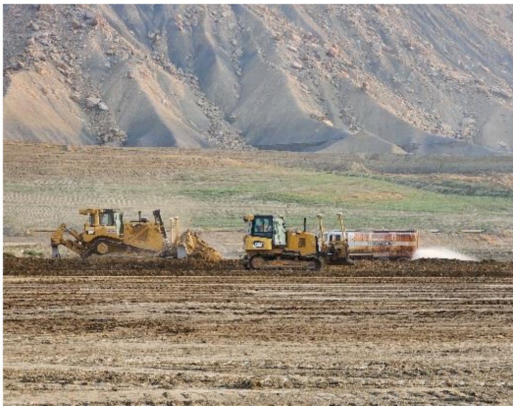
Photo 28. Water truck moisture conditioning; D6& D8 dozer placing Manco Shale July 2024
