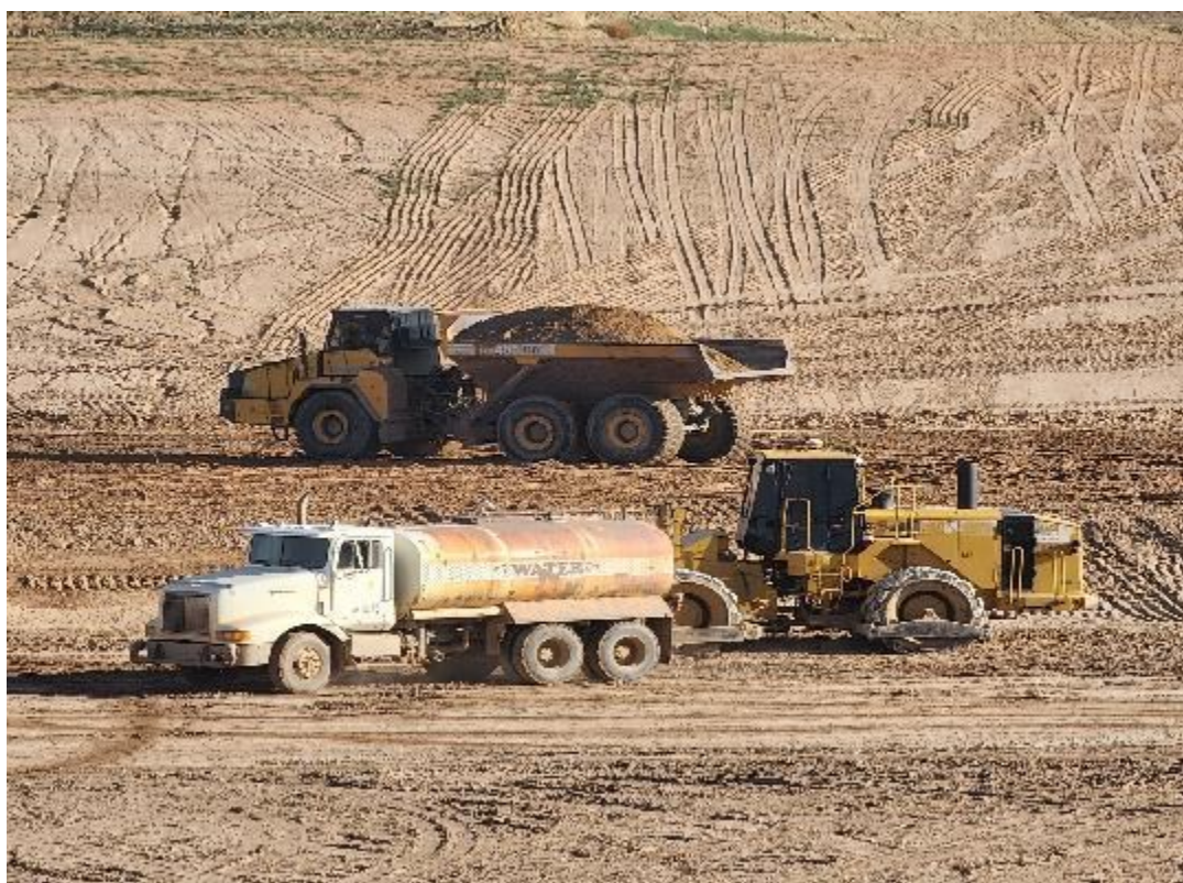
Photo 18. Compactor, water truck, and haul truck working together June 2024
