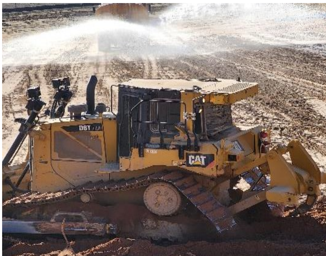
Photo 6. Water truck moisture conditioning lift December 2023
