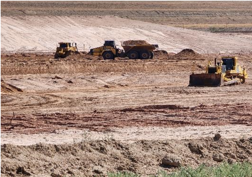
Photo 20. Haul truck getting ready to unload RRM for dozer to place July 2024
