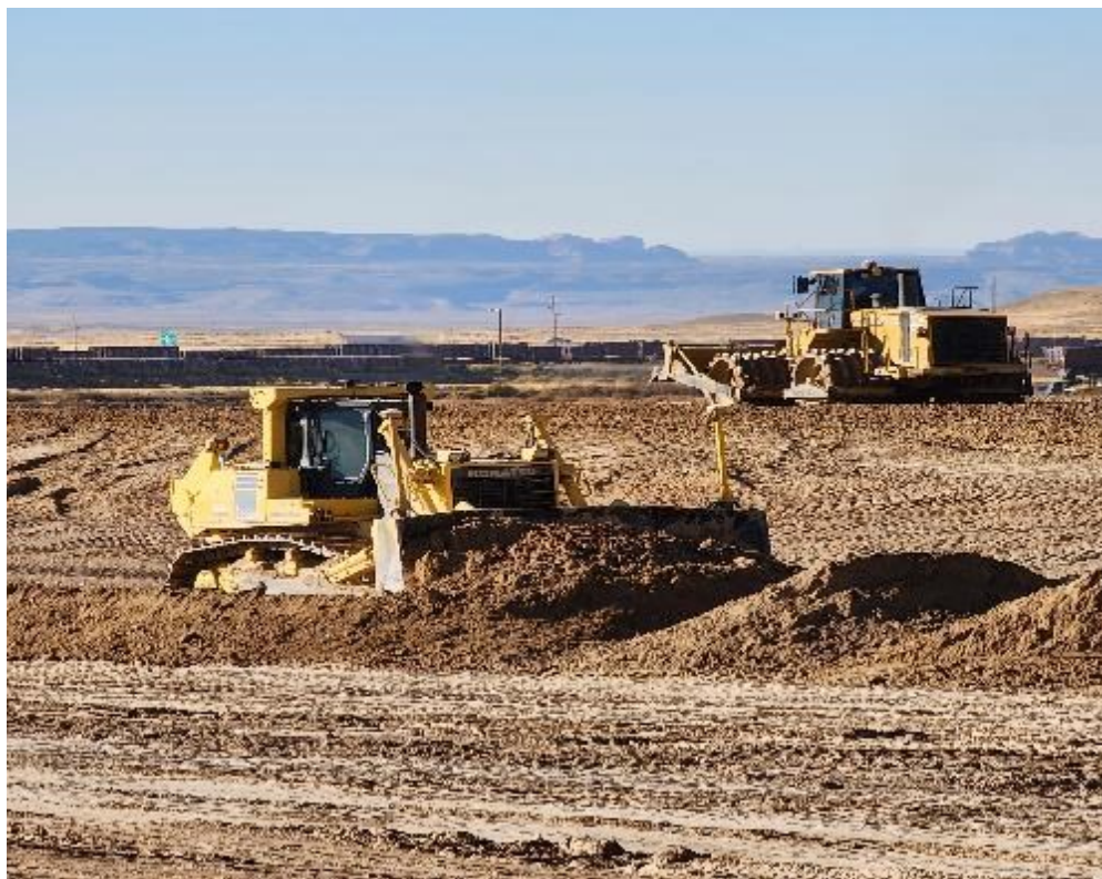
Photo 1. Dozer placing RRM and compactor compacting on lift above October 2023
