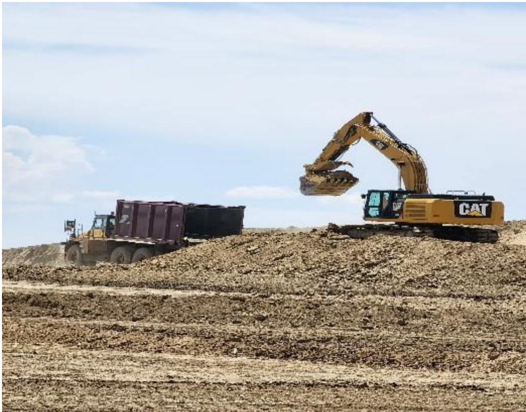
Photo 30. Loading protective cover for Interim cover August 2024
