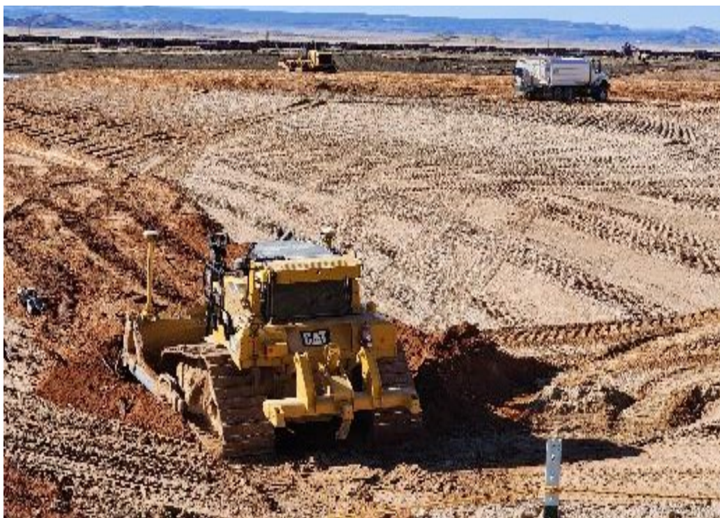
Photo 11. Dozer placing debris/RRM mix March 2024
