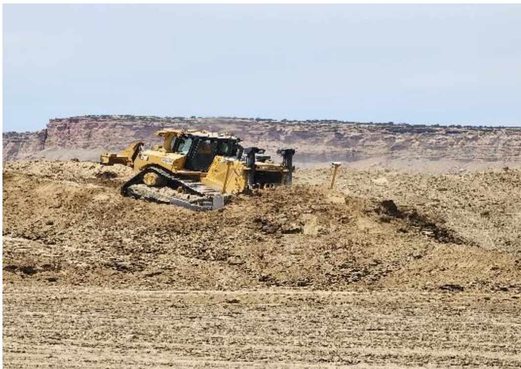
Photo 26. Pushing Manco Shale for Interim Cover July 2024
