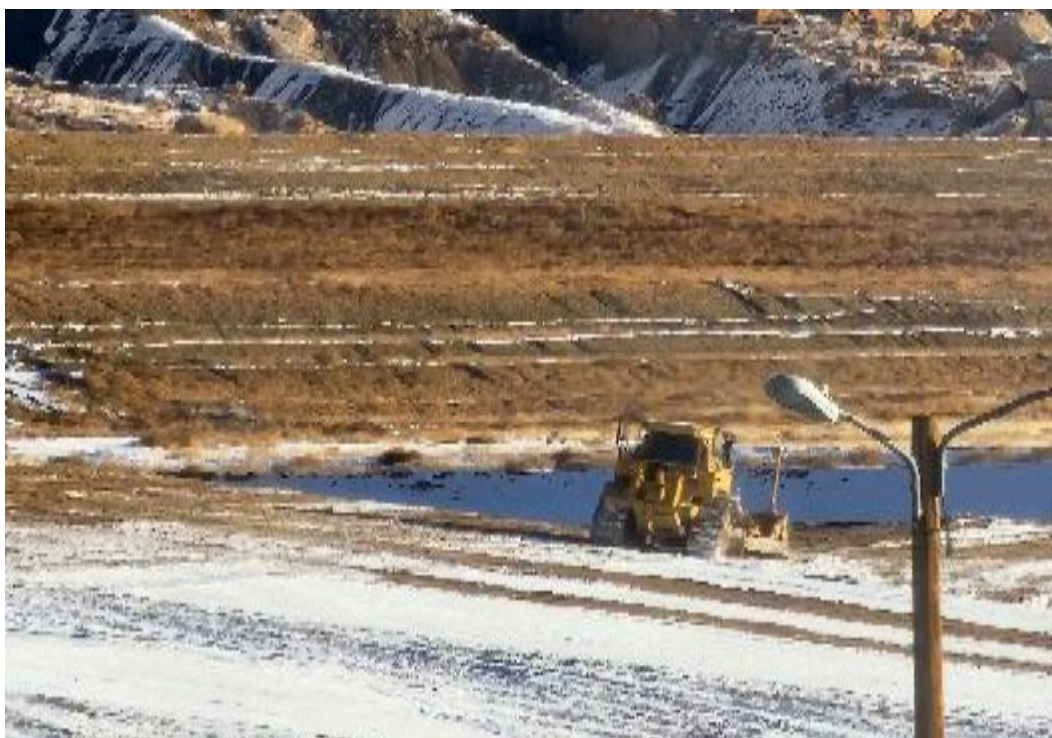
Photo 8. Cleaning snow of the lift before placement January 2024
