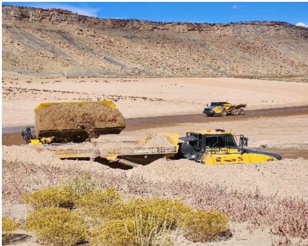
Photo 2. Loader loading RRM into haul truck in cell October 2023
