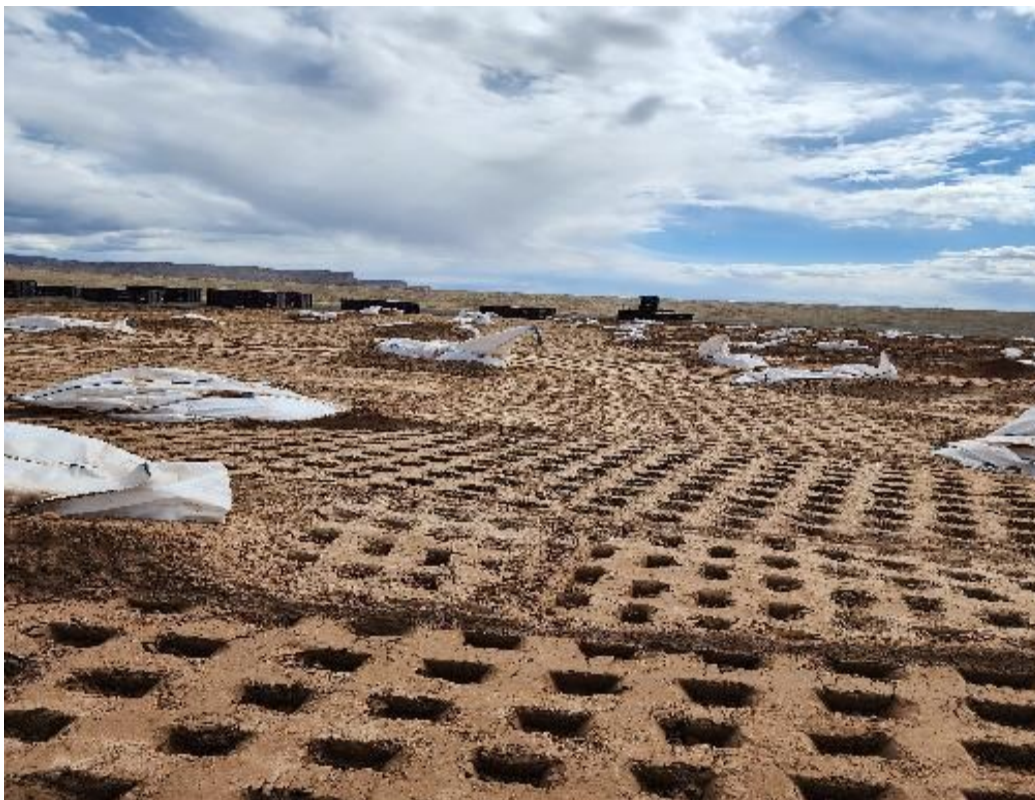
Photo 13. Compaction between asbestos sacks April 2024
