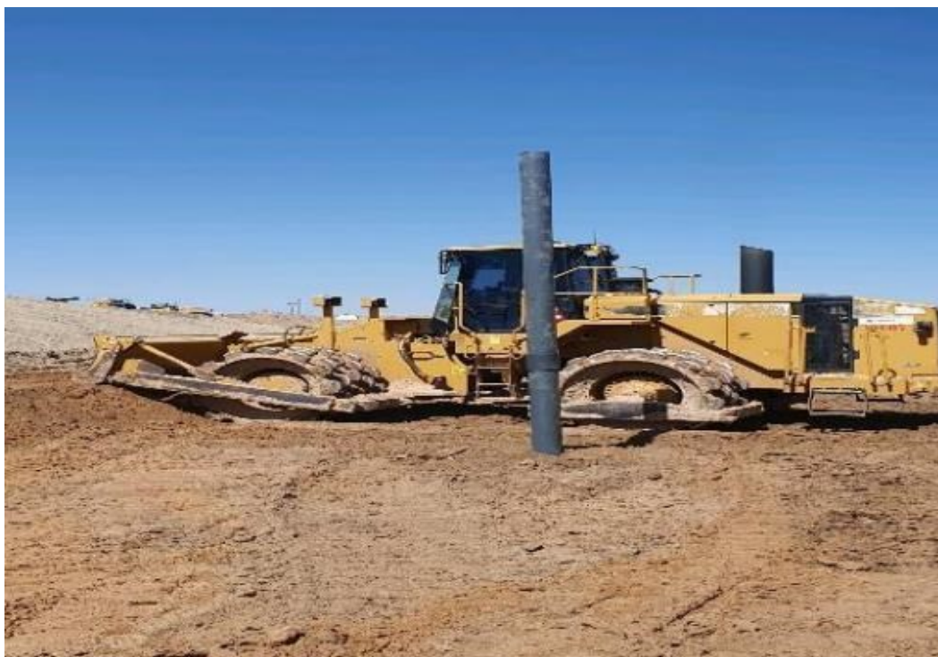
Photo 27. Compacting around standpipe. May 2023
