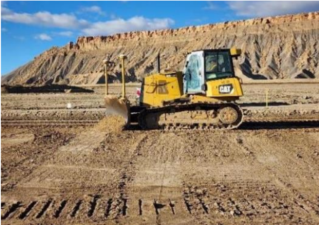
Photo 41. Grading Interim cover. November 2022
