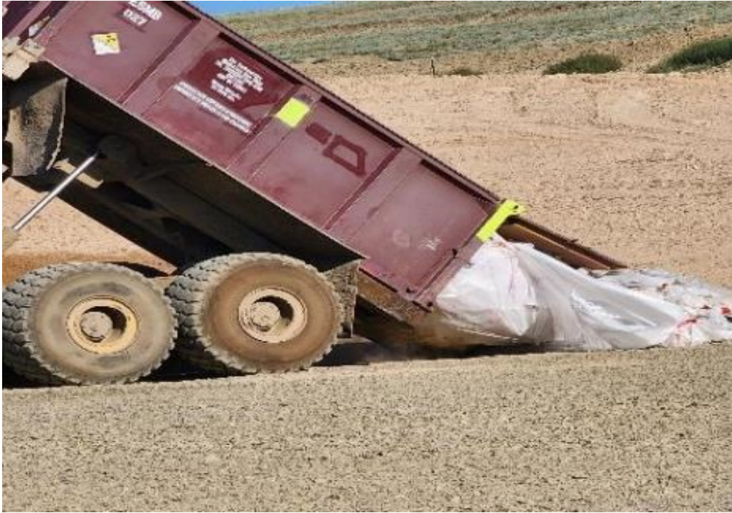
Photo 31. Dumping asbestos sacks in cell. July 2023
