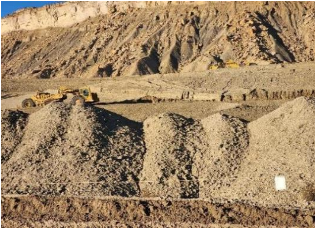
Photo 58. Scrapers hauling to top of spoils November 2022
