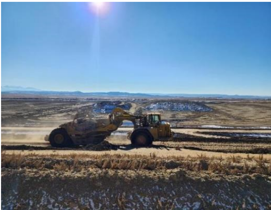
Photo 59. Scraper placing on spoils loop December 2022
