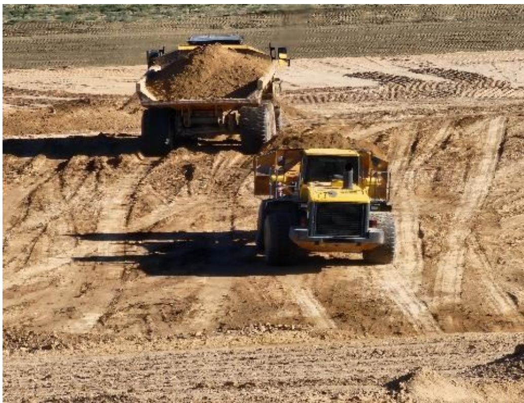
Photo 29. Truck & loader hauling RRM to lift. June 2023
