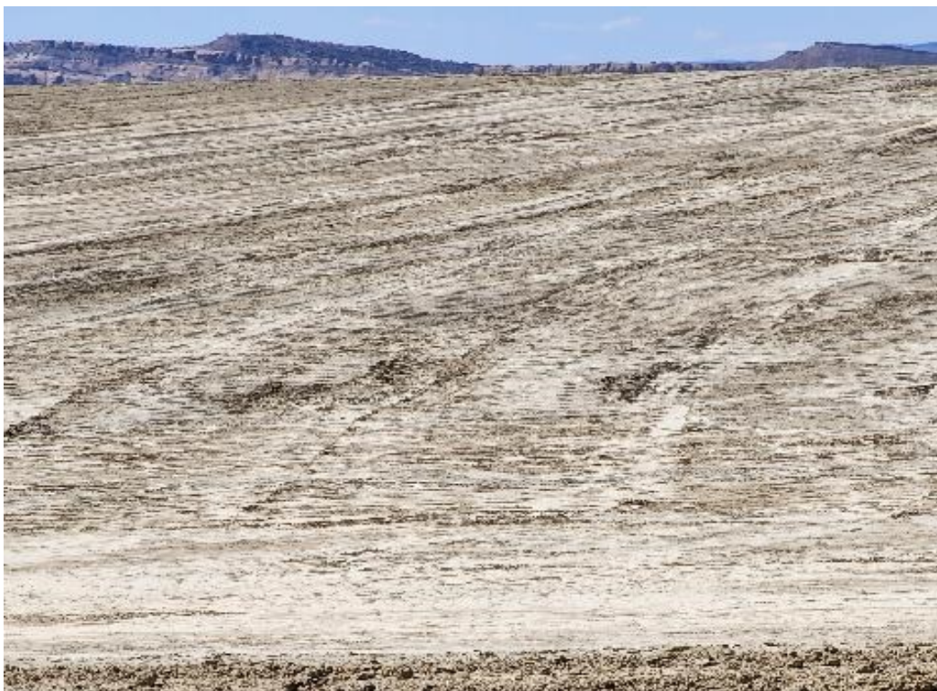
Photo 55. Radon Barrier completed. June 2023
