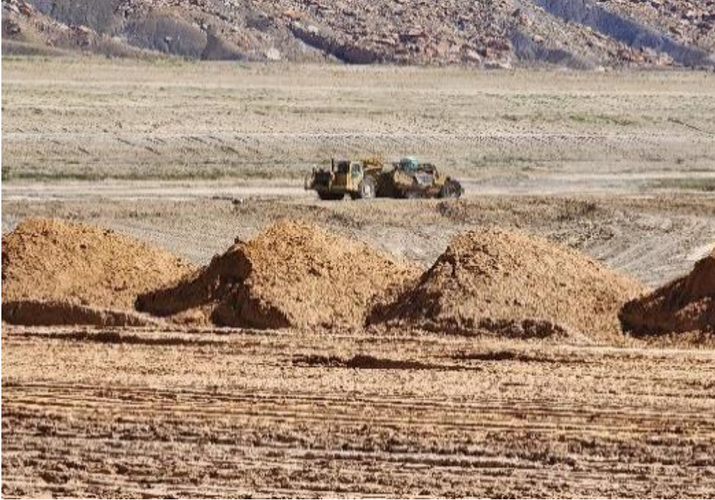
Photo 53 Scraper hauling to radon barrier May 2023
