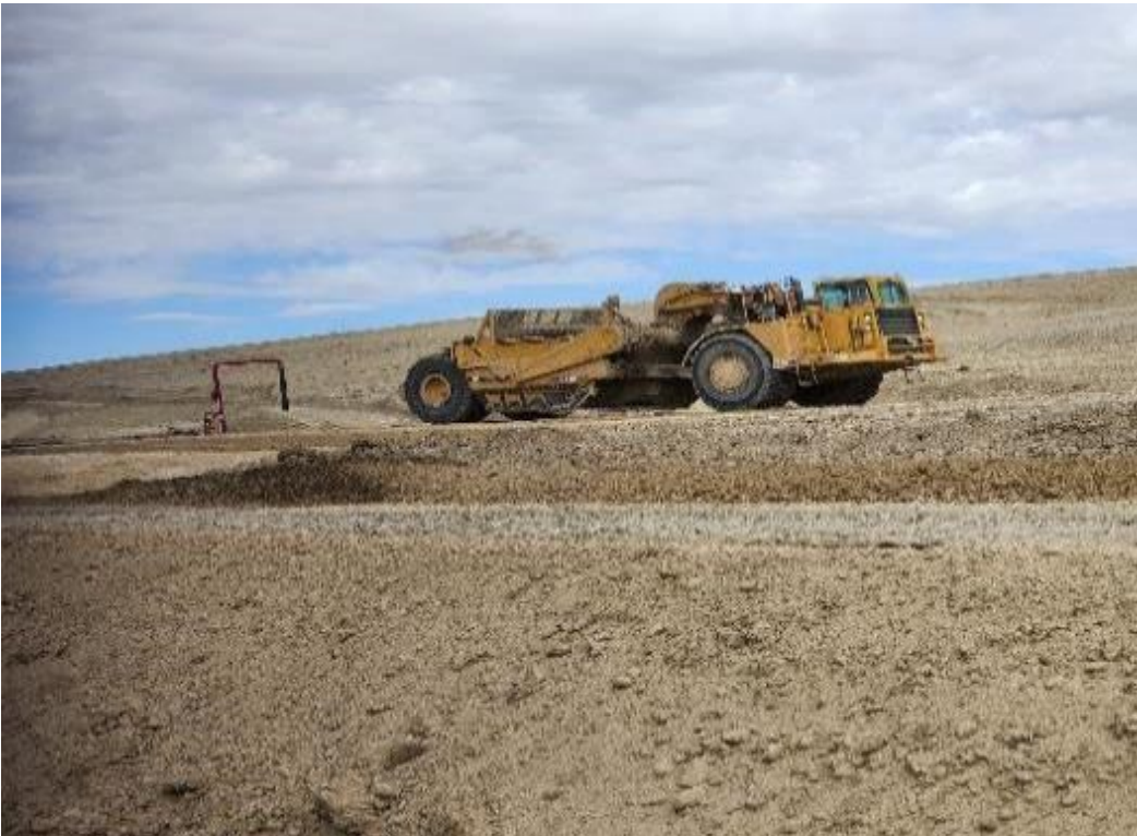
Photo 54. Scraper hauling on stockpile May 2023
