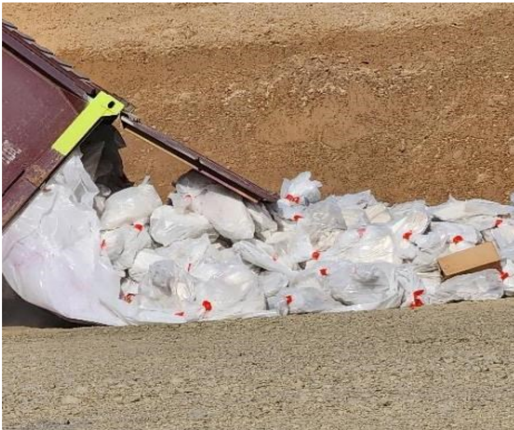
Photo 32. Disposal of asbestos sacks in cell. July 2023
