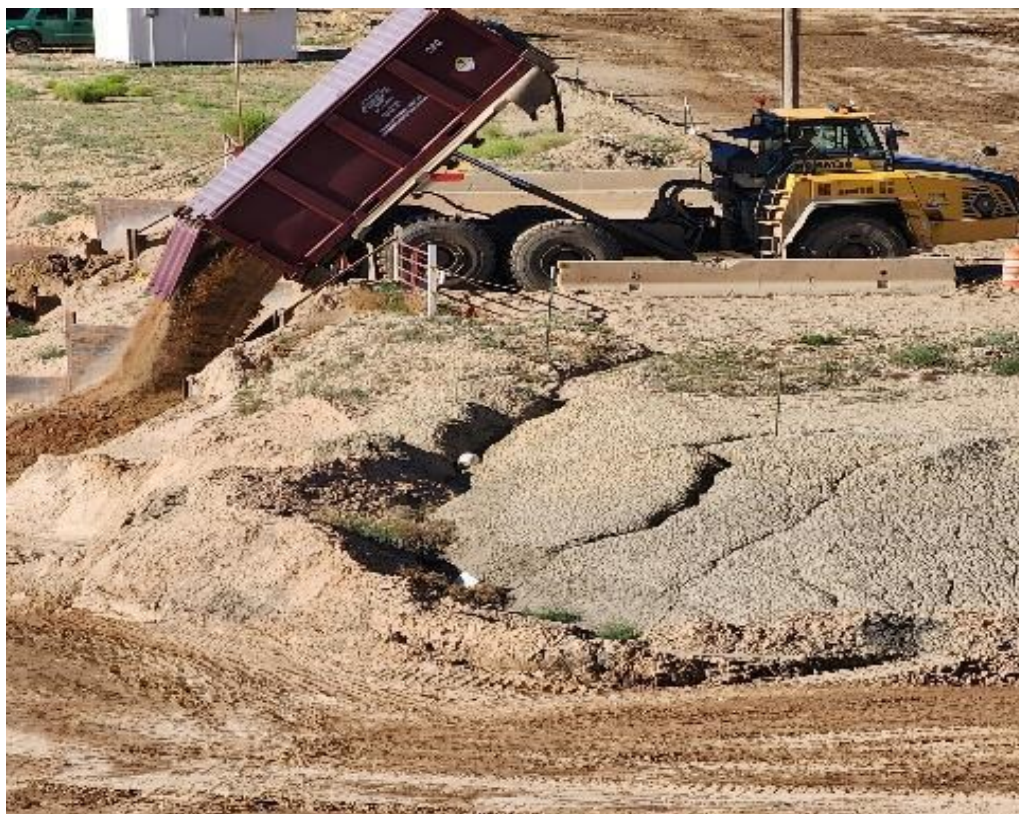
Photo 30. Unloading RRM into cell. June 2023
