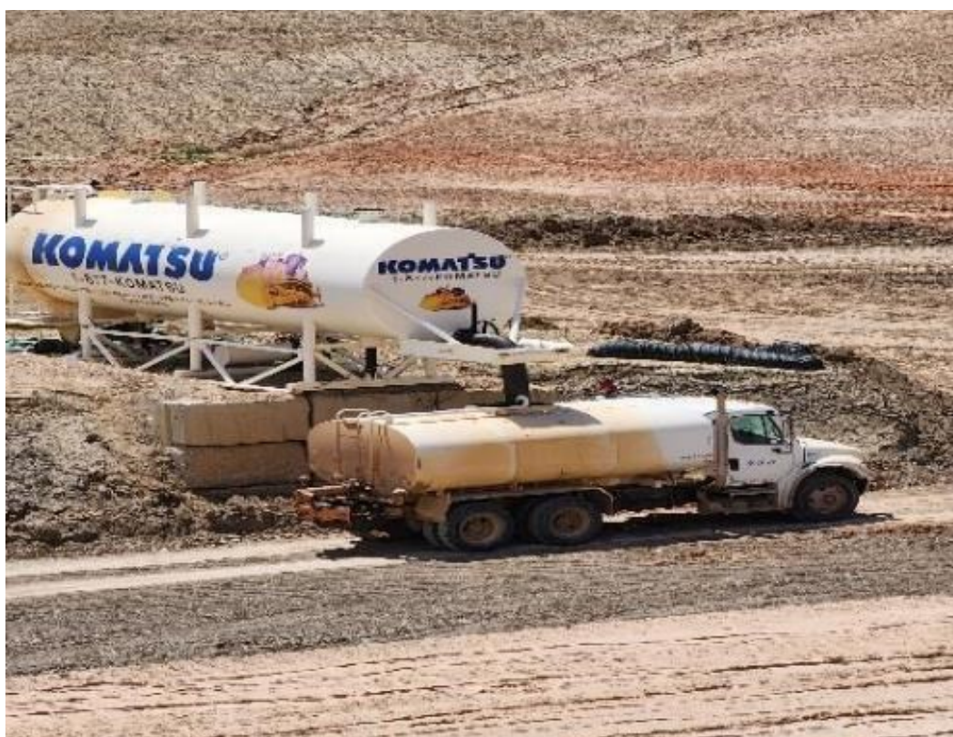
Photo 28. Water truck filling for dust control. May 2023
