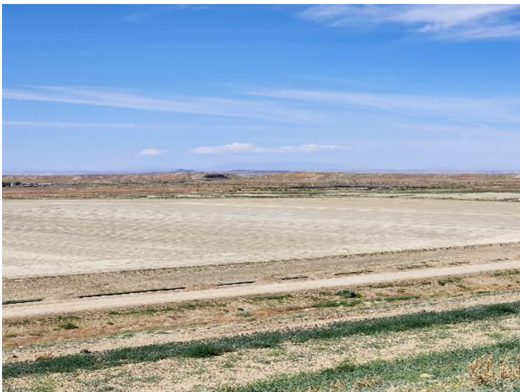
Photo 56. Radon Barrier completed and smooth drum rolled. June 2023
