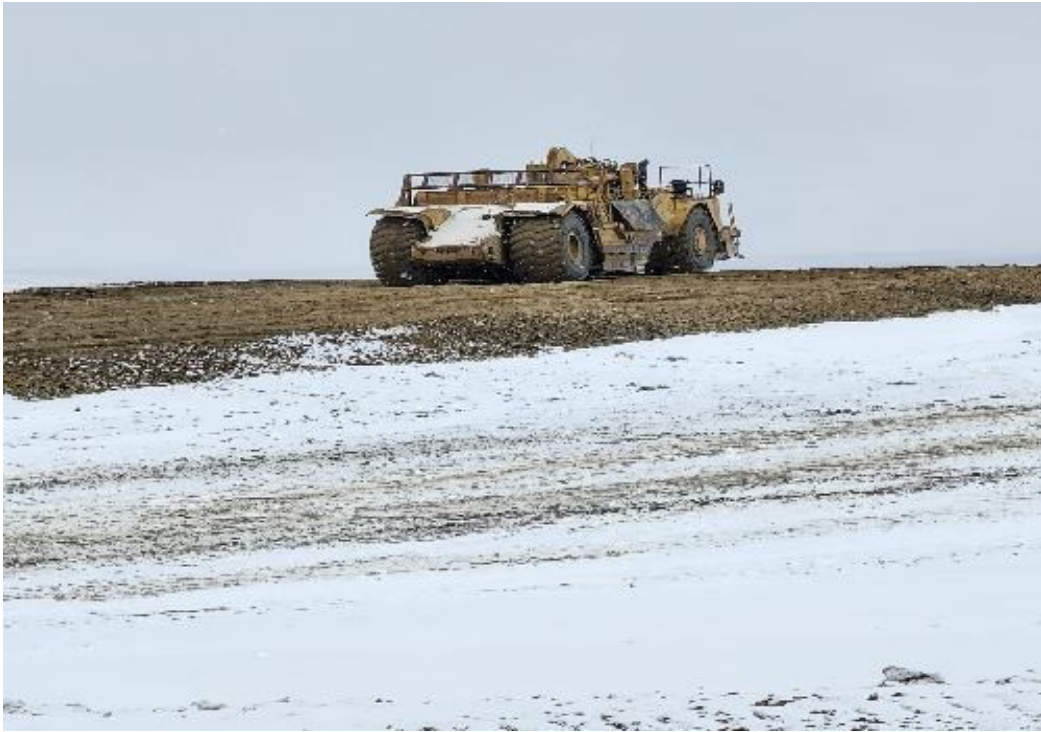
Photo 47. Scraper placing Mancos Shale. February 2023
