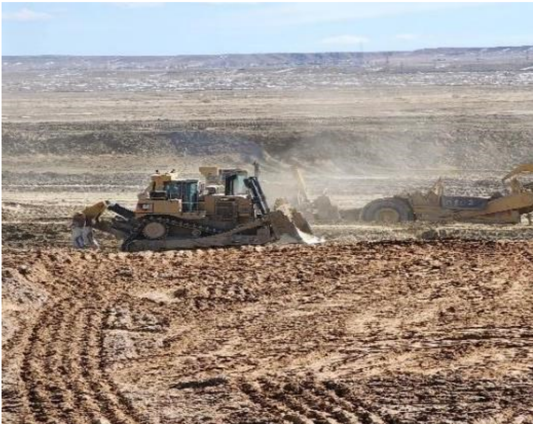
Photo 6. Ripping Mancos Shale with dozer March 2023
