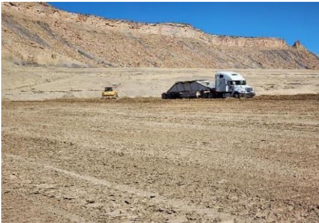
Photo 39. Spreading and placing Interim cover. October 2022
