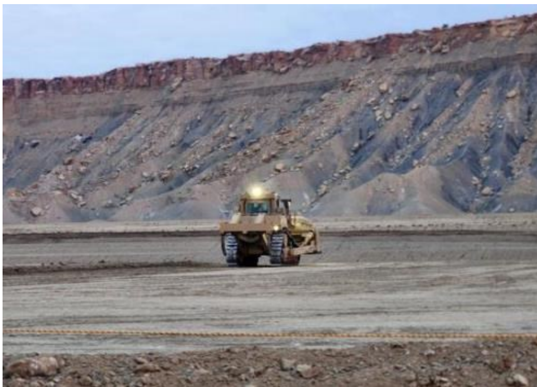
Photo 43. Ames tracking radon barrier. December 2022
