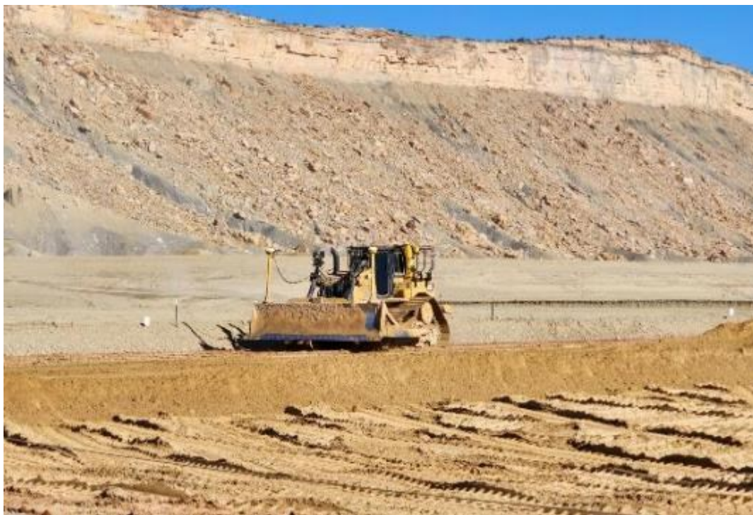
Photo 17. Placing RRM for Top of Waste December 2022
