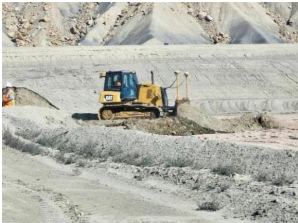
Photo 40. Pushing Interim cover over TOW. October 2022
