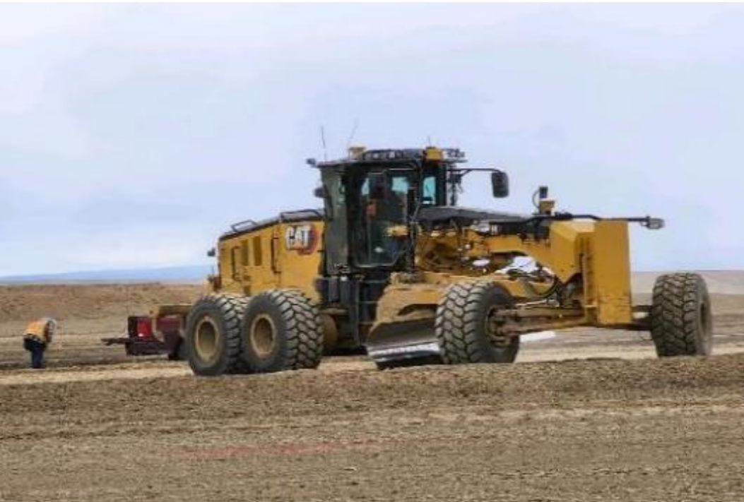
Photo 52. Ames grading radon barrier. April 2023
