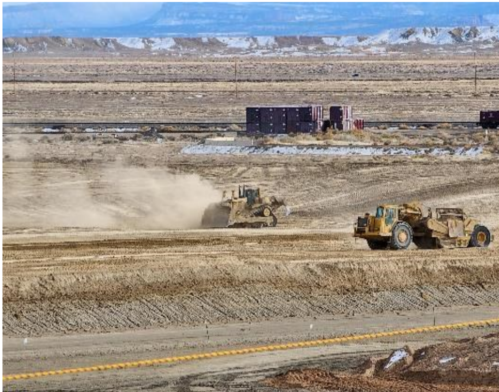
Photo 2. Dozer pushing cell floor December 2022
