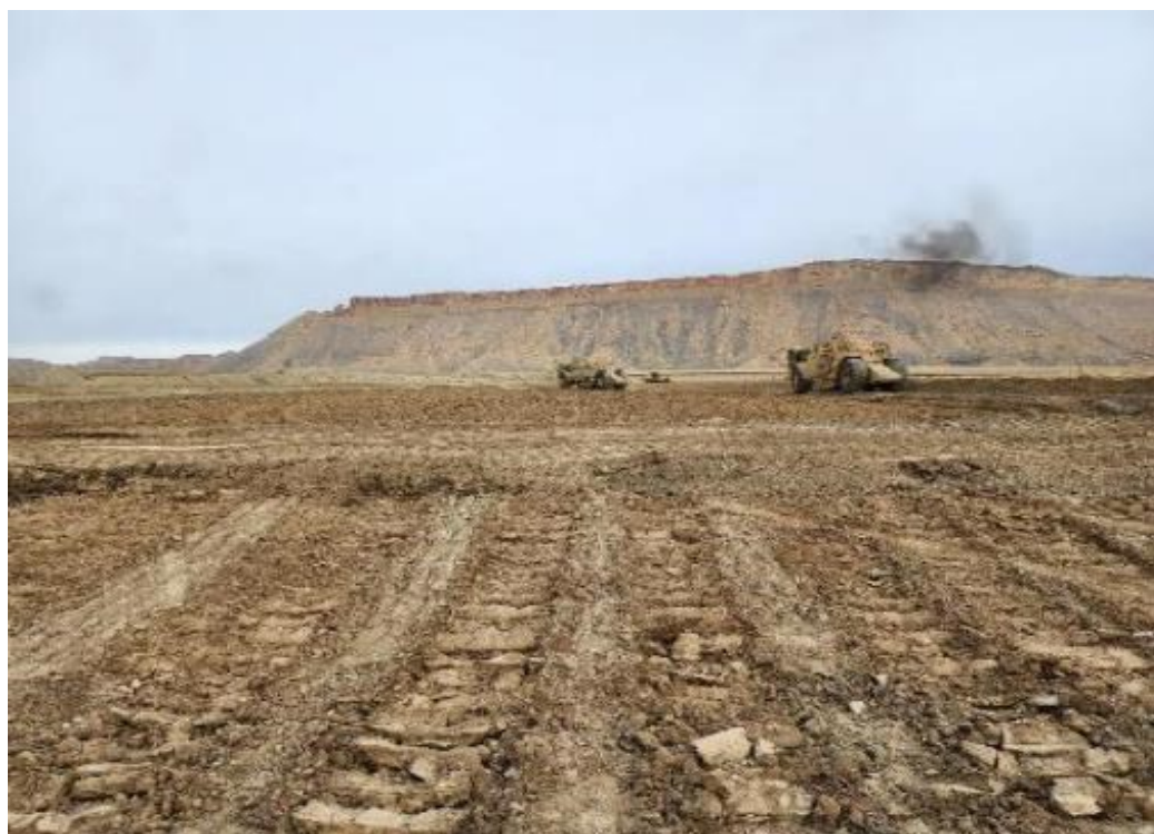
Photo 44. Ames placing Mancos Shale on Radon Barrier lift. December 2022
