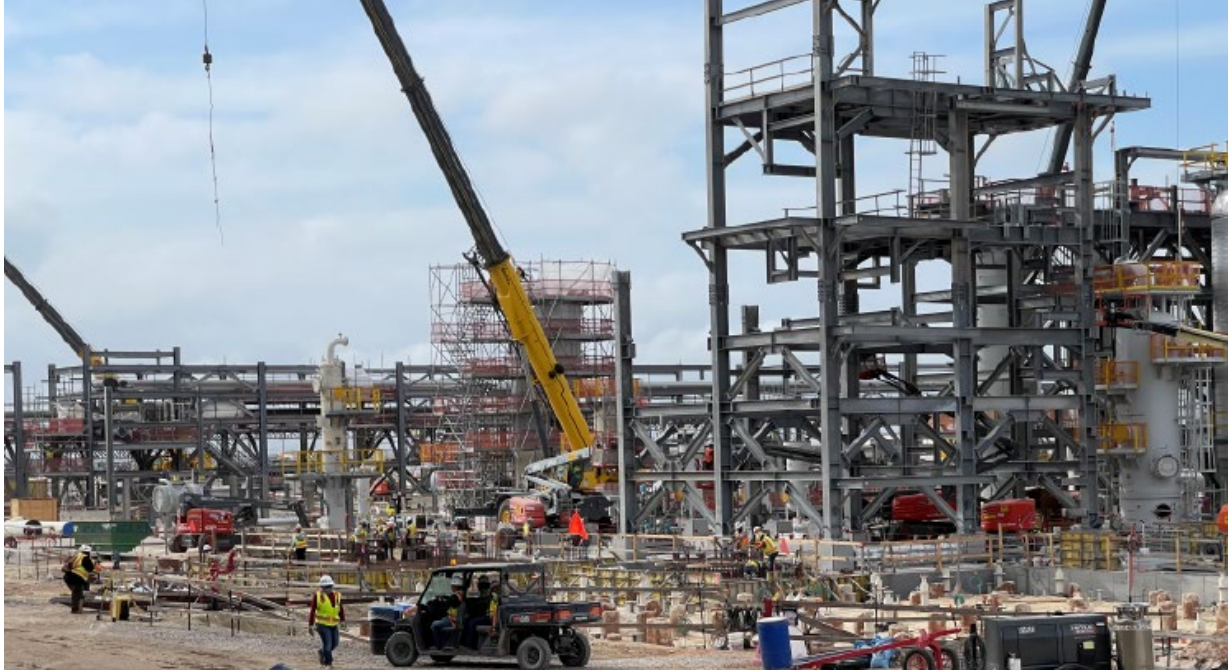
Photo 3: Train 5 Structural Steel
