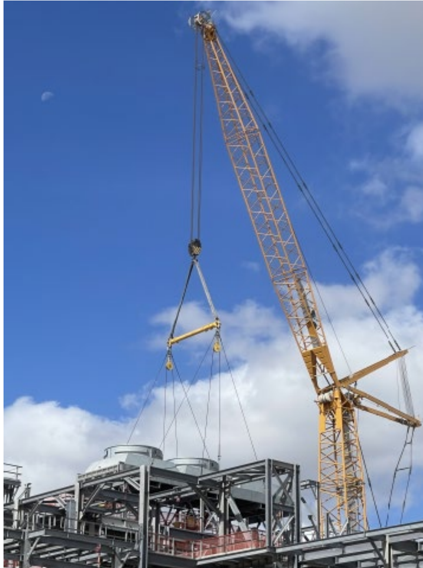
Photo 1: Train 4 Air-Cooled Heat Exchanger Installation
