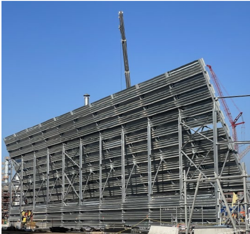
Photo 5: Flare 2 Heat Shield Erection
