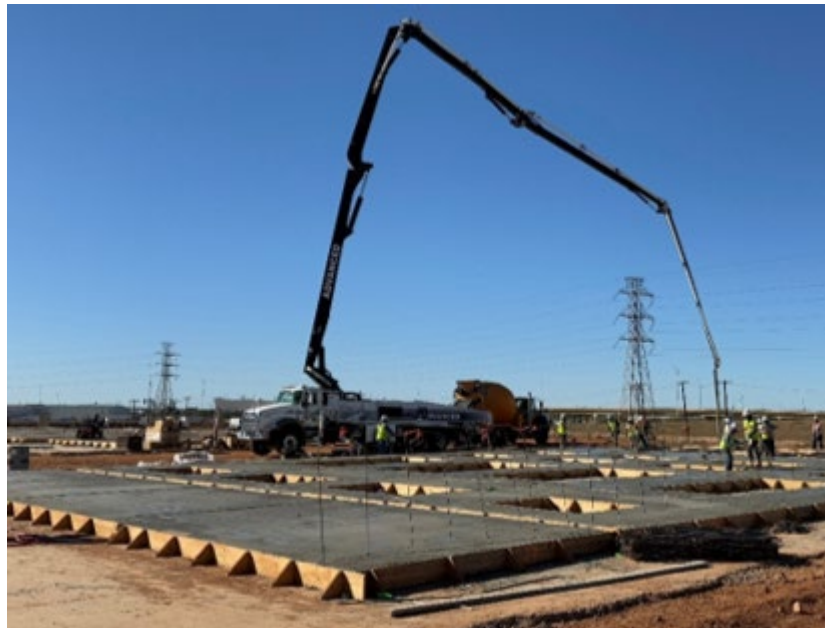
Photo 4: O&M Building Concrete Placement
