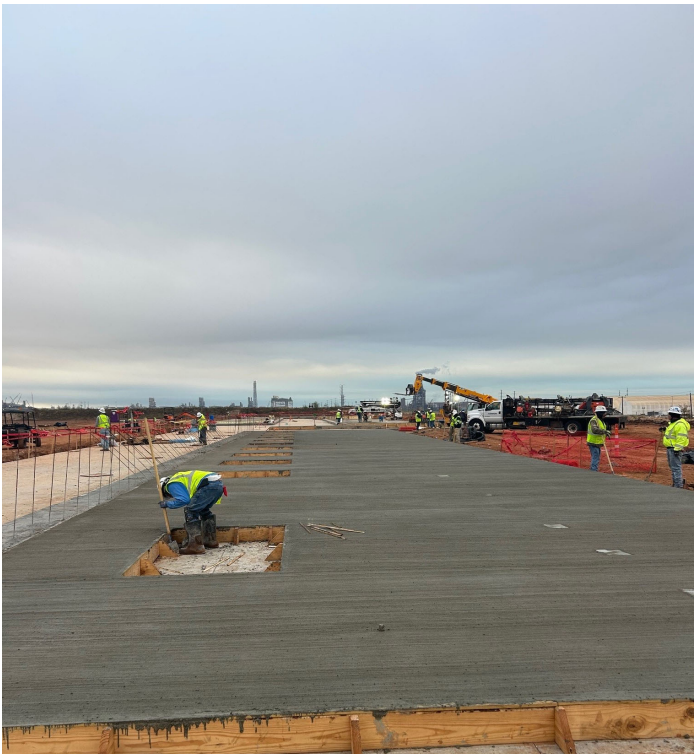
Photo 5: O&M Building Concrete Placement
