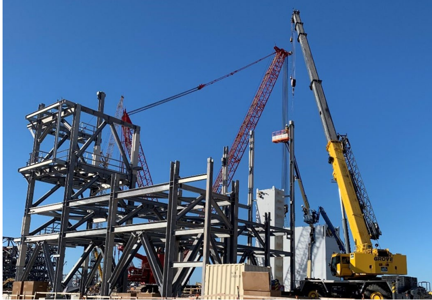
Photo 4: Train 6 Structural Steel Installation
