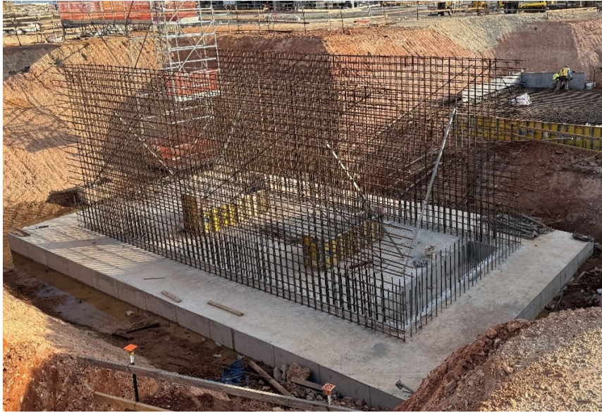
Photo 1: Train 6 Amine Sump Foundation
