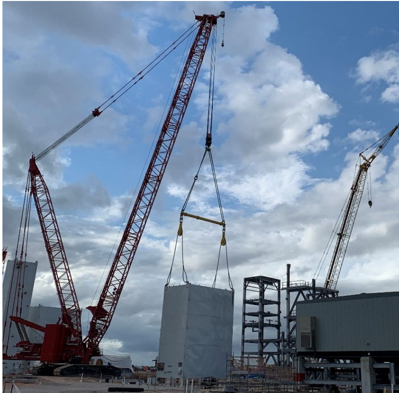
Photo 2: Train 6 Cold Box Installation
