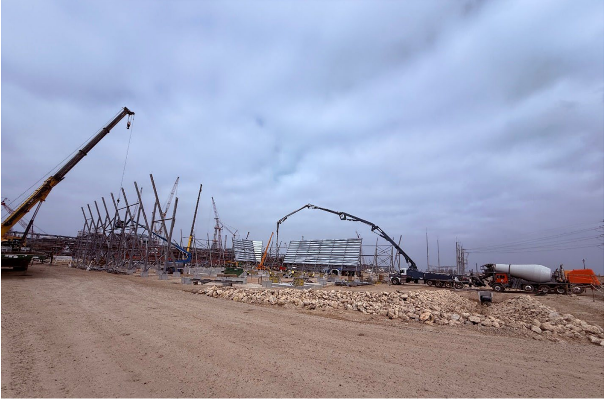
Photo 5: Ground Flare No. 3 Structural Steel
