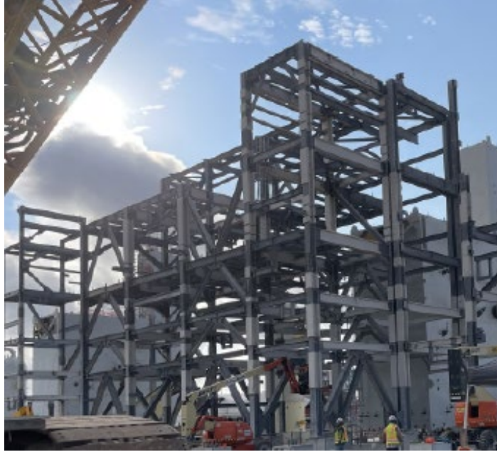
Photo 3: Train 5 Cryo Rack Structural Steel Installation
