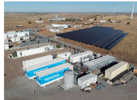
The ARIES facility Large scale H 2 production and power generation; available for H 2 release studies (commissioned in January 2024).
