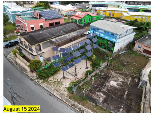
Figure 2: New microgrid sponsored by project, will serve 7 residences, allow networked operation, and be a space for workforce development. Planned completion, December 2024.
