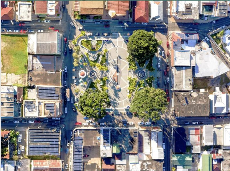
The community of Adjuntas, in central Puerto Rico, is aiming to become an all-solar town. CASA PUEBLO
