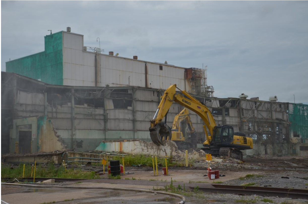
Figure 3.1. D&D of the C-410/C-420 Feed Plant Complex
