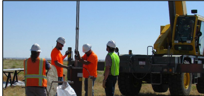
Maintenance personnel performing a pump replacement at a monitoring well
