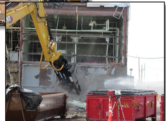
Demolition in progress for S1W diesel generator and radiac calibration rooms
