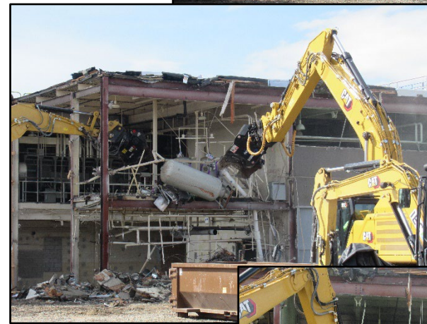
Demolition in progress for S1W diesel generator and radiac calibration rooms
