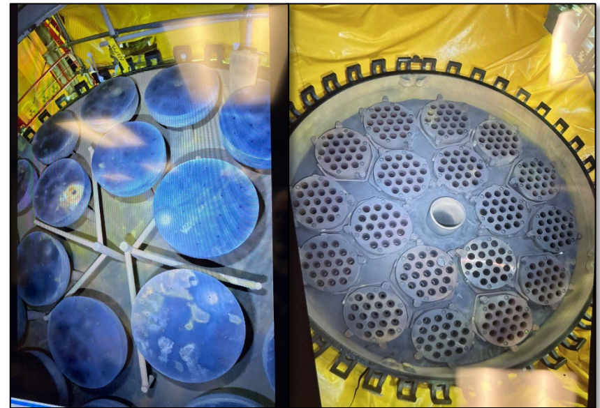
Views of PGF vessel head & tubesheet during remote inspection
