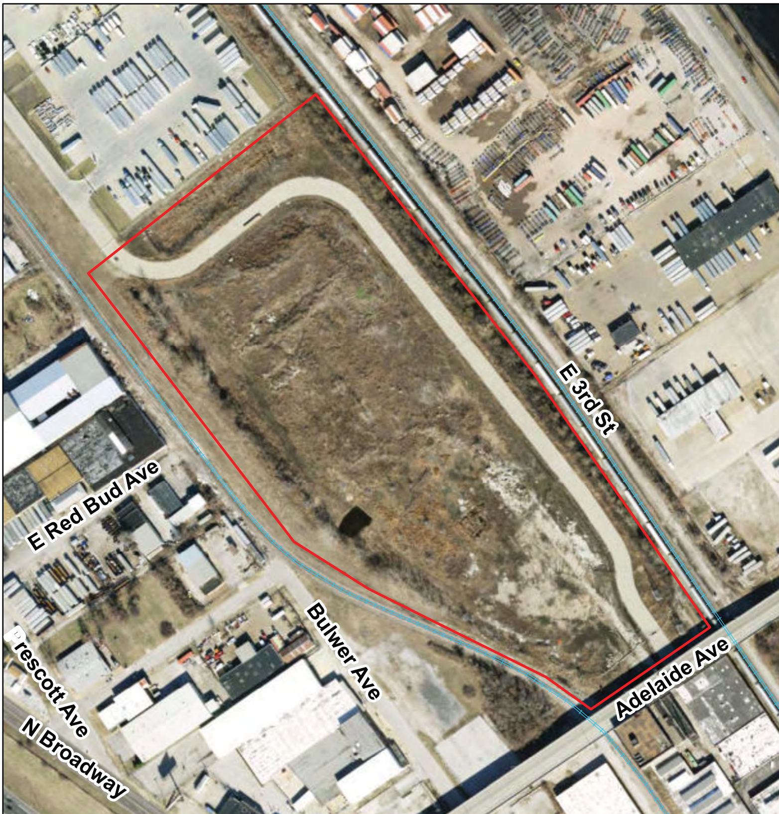
Figure 2. Aerial View of Proposed Project Site
