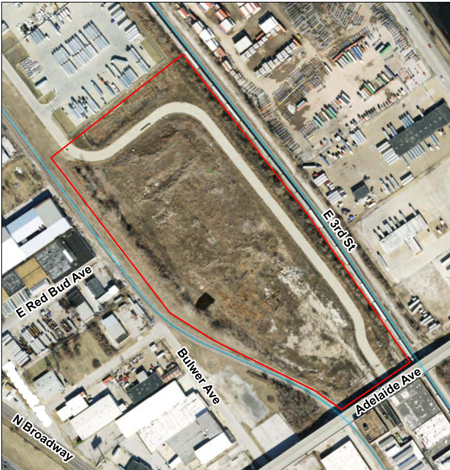
Figure 2. Aerial View of Proposed Project Site
