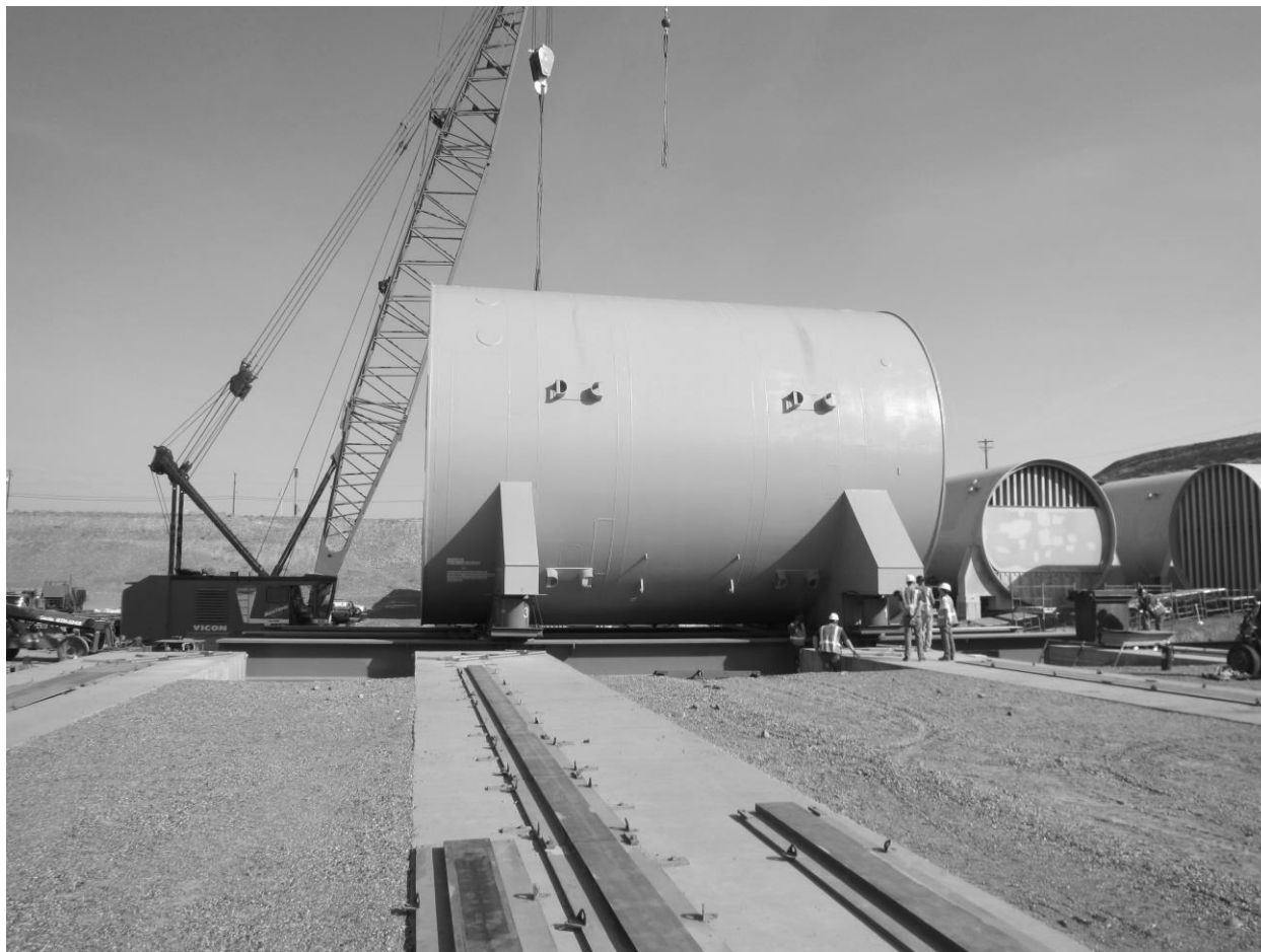
Preparing to move a Reactor Compartment Package into place on the Rail Delivery System in the Disposal Trench at Hanford
