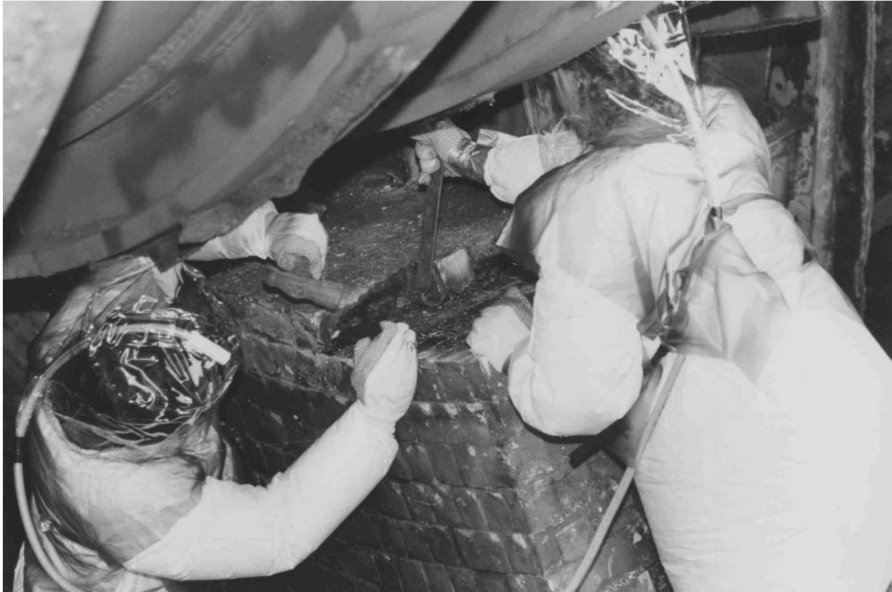
Lead Ballast Removal
