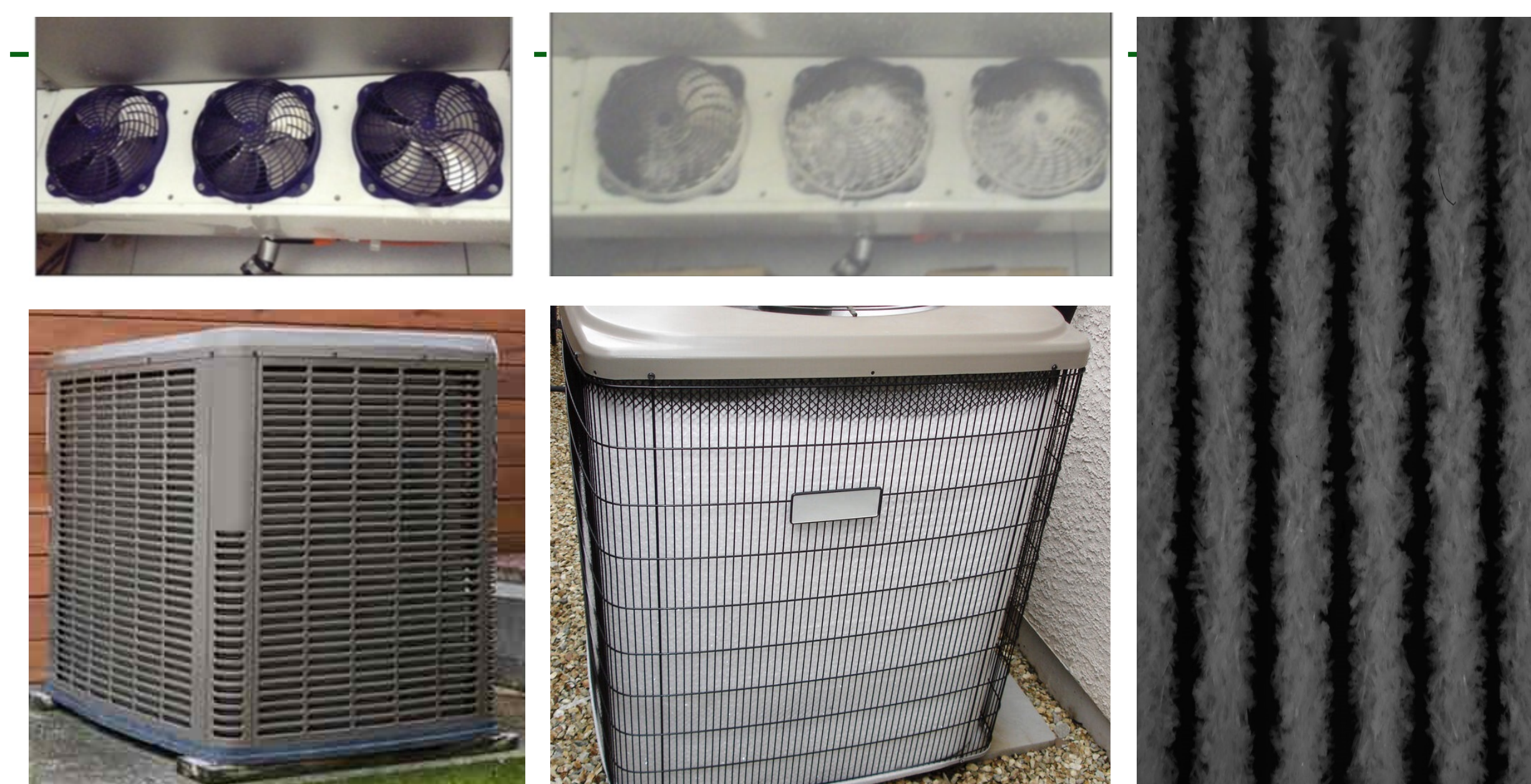
Frost buildup in a walk-in freezer and cold climate heat pumps
