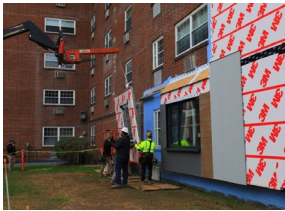
Envelope Improvement (Prefab Unitized Panel)
