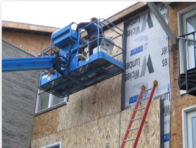
Using Retrofit Nail Base Panels to improve insulation in the building envelope
