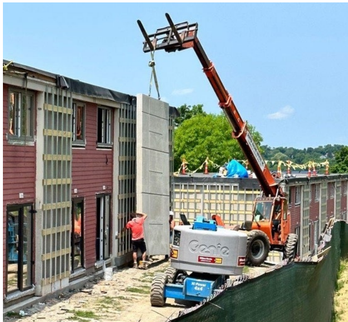
Prefabricated exterior panel installation
