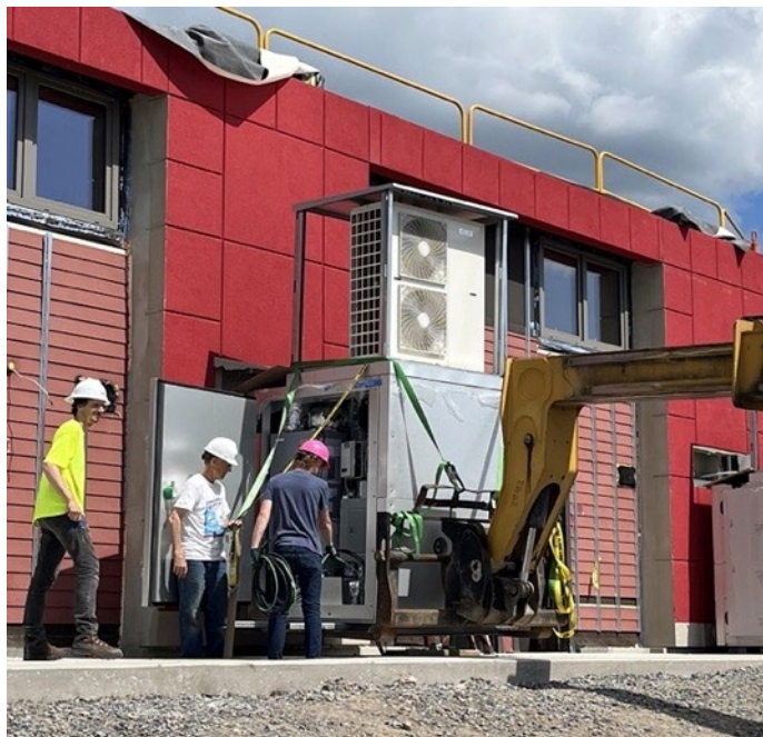
TKFabricate mechanical pod installation
