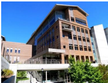
UC Berkeley Sutardja Dai Hall Large Commercial Building Streamlined Controls Deployment
