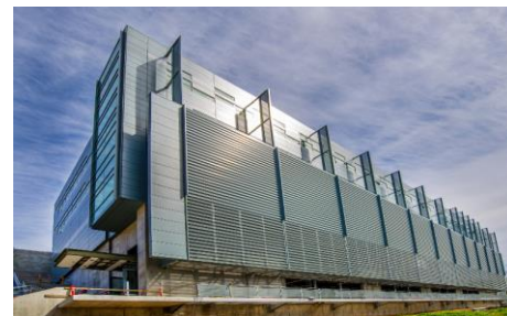
LBNL Building 59 Large Commercial Building Automated Large Building MPC
