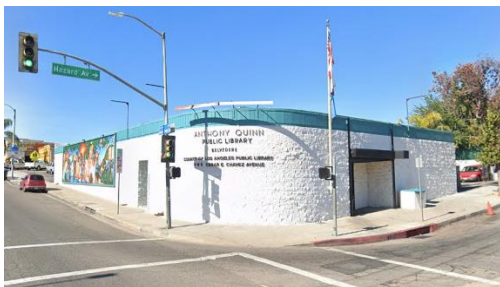
Anthony Quinn Library Small Commercial Building Application-Driven Modeling + MPC
