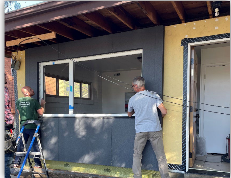
First panels with window cassettes installed on first building. (Photo courtesy Michele Knapp, FunForm)
