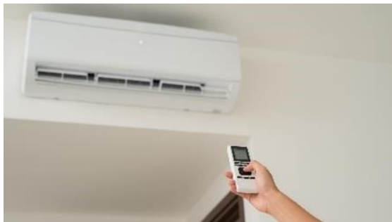
Mini-split heat pump inside head unit. Image from Building America Solution Center.
