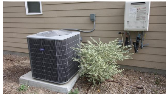
Ducted heat pump outside compressor. Image from Building America Solution Center.
