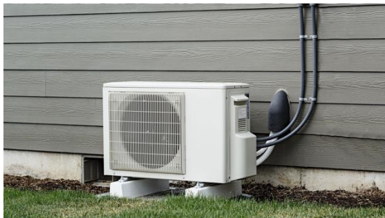
Ductless heat pump outside compressor. Image from Building America Solution Center.
