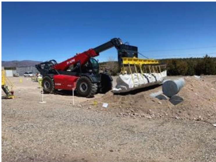
Surrogate CMP in an IP-1 bag being retrieved from excavation using spreader beam and the Telehandler
