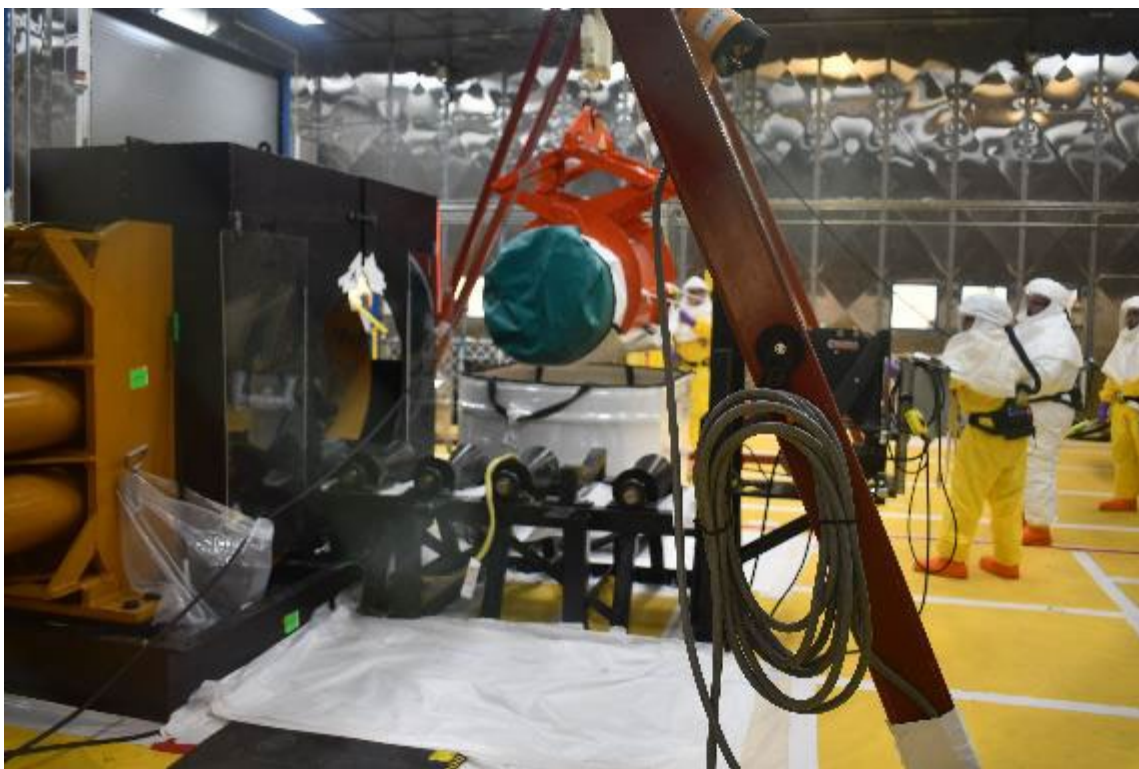
Placement of a cut CMP section into a Standard Waste Box
