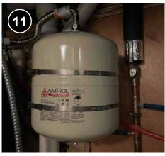
Support the expansion tank so thatit does not move or sag using rigid support material that is able to supporttwice its weight when filled with water. 7.0303.5d.
