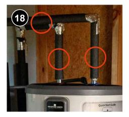
On all accessible pipes carrying hot water, install pipe insulation of R-3 or better that is a vapor retarder and sized for the correct diameter of the pipes. 7.0301.1b.
