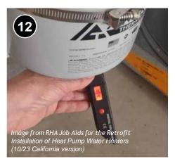
Set the pressure in the expansion tank to match incoming water pressure. 7.0303.5e.
