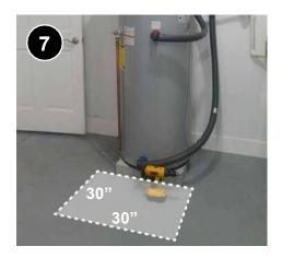
Double check clearance in front of the unit's control side to allow at least 30" x 30" to allow for inspection, maintenance, and replacement of components. 7.0302.3e.
