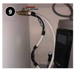
If not already present, install separate water cut-off valves for both hot- and cold-water lines. 7.0302.3h.
