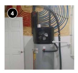
Ensure the room meets requirements for the unit. Is there enough volume and clearance for airflow around the unit? Are the ceilings high enough? Is there adequate space to allow maintenance of the heat pump components, including removal and cleaning of the air filter? Ensure the unit will not blow directly on an indoor thermostat or occupants. 7.0302.3c.
