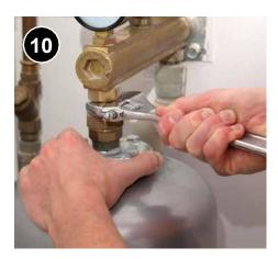
If the cold water supplying the HPWH passes through a check valve, pressure reducing valve (PRV), or backflow preventer, install an expansion tank on the cold- water supply line at a point that is downstream of all those valves. Size the expansion tank in accordance with manufacturer specifications and applicable code. 7.0302.3i.
