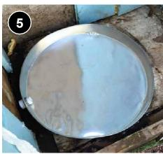
If the HPWH will be installed in or above conditioned space or in a location where water damage could occur, install a drain pan according to IRC requirements. Drain the pan to the exterior of the building. 7.0302.3g.
