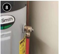
Install a Temperature and Pressure (T&P) relief valve per IRC and manufacturer specifications. Pipe the valve to within 6" of the floor or drain pan, or directly to the outdoors in an observable location. Piping material must meet IRC requirements. 7.0302.3f.
