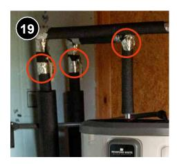
Seal all insulation seams, joints, and connections with tape, tie straps, or other independent means. 7.0301.1c.
