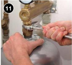
If the cold-water supply passes througha check valve, pressure reducing valve (PRV), or backflow preventer, install an expansion tank on the cold-water supply line at a point that is downstream of all those valves. Size the expansion tank in accordance with manufacturer specifications and applicable code. 7.0302.6I.
