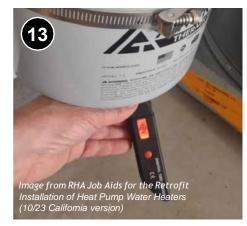
Set the pressure in the expansion tank to match incoming water pressure. **7.0303.5e**.
