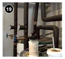
On all accessible pipes carrying hot water, install pipe insulation of R-3 or better that is a vapor retarder and sized for the correct diameter of the pipes. 7.0302.6m.
