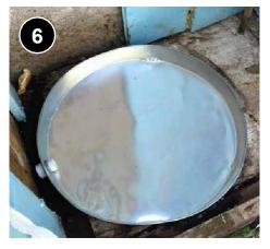
If the storage tank will be installed in or above conditioned space or in a location where water damage could occur, install a drain pan according to IRC requirements. Drain the pan to the exterior of the building. **7.0302.6g**.
