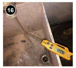
Set the discharge temperature to 120°F. Install temperatureindicating device at the discharge outlet of the thermostatic mixing valve. 7.0302.6n.
