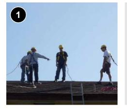
Verify the plumbing infrastructure is leak-free and sufficient to support a solar hot water installation. If mounting the solar collector on the roof, verify the roof will adequately support the installation (dead load and wind load) and that the roof has more than 10 years of useful life remaining. Consider using Weatherization Readiness Funds (WRF) if this is not the case. 7.0302.6a.
