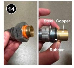
Install dielectric unions when connecting copper to galvanized steel piping in accordance with IRC and manufacturer specifications. **7.0302.6i**.
