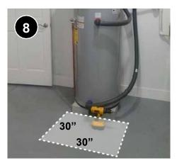
Double check clearance in front of the storage tank to allow for inspection, maintenance, and replacement of components (including replacement of the anode rod). 7.0302.6e.
