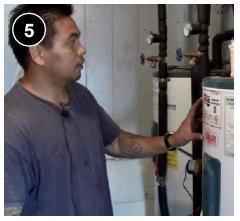
Select a storage tank/backup water heater that is ENERGY STAR<sup>®</sup> certified, equivalent, or better; fits in the installation space with required clearances; provides sufficient hot water for the home and occupants; and is insulated to R-12.5 or greater. **7.0302.6b**.
