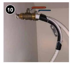
If not already present, install a separate water cut-off valve for each incoming water line at the storage tank, and between each additional component of the system (e.g., mixing valves, solar collector, additional storage tank). 7.0302.6k.
