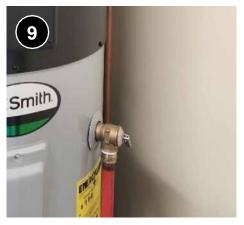
Install a Temperature and Pressure (T&P) relief valve per IRC and manufacturer specifications. Pipe the valve to within 6" of the floor or drain pan, or directly to the outdoors in an observable location. Piping material must meet IRC requirements. **7.0302.6h**.
