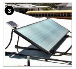
Locate solar collectors to minimize shading and maximize solar gain without interfering with other appliance operations (e.g., chimneys, vents, and exhaust terminations). 7.0302.6c.
