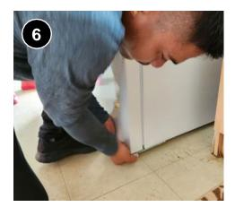
Use a level to check for level left to right. It's best to use the frame of the refrigerator itself. Adjust the refrigerator feet if necessary. Ensure the appliance does not reduce required maneuvering clearances in the kitchen to less than those permitted by local, state, or federal guidelines. 70101.1d.
