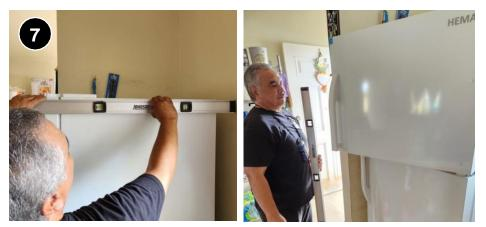
Now check for level front to back, again using the frame of the refrigerator. You will want the unit to lean slightly to the rear, so the door gently closes on its own. Adjust the feet if necessary.
