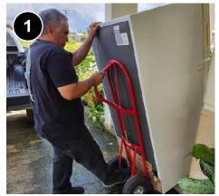
Unplug and remove the old refrigerator from the home, taking care to avoid damaging walls, floors,doorways, etc. Verify the electrical receptacle meets the requirements of NFPA 70 Article 422 (Maximum breaker size for the circuit matches the breaker marking on the appliance).
