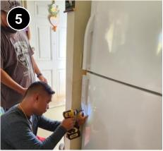
Move the new refrigerator into place and install appliance according to manufacturer specifications and applicable code. If a water line is present, connect the line to the new refrigerator being careful not to damage the line or fittings. Turnthe water on and check for leaks. At this time, you may also need to install handles and shelving per manufacturer instructions. **7.0101.1c.**
