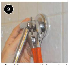
Carefully remove old showerhead with adjustable wrench, taking care not to loosen shower arm.
