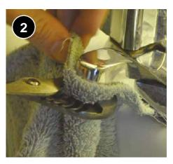
Using adjustable wrench or aerator wrench, gently remove old aerator, taking care not to damage faucet.
