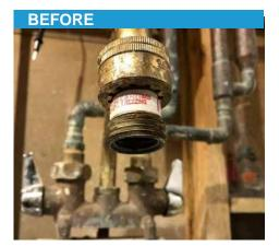
Faucets without aerators produce excess flow and old aerators can impinge flow or cause leakage.
