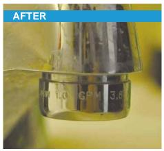
Low-flow faucet aerators limit flow to 2.2 gallons per minute or less and reduce water heating load by reducing water usage. **7.0201.1b.**
