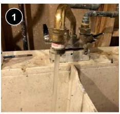
Verify current plumbing infrastructure is sufficient to support the installation(s) and water is free of visible debris that may clog the equipment. 7.0201.1a.
