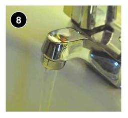
Run water through new aerator to verify it is not cross-threaded and no water is leaking around sides.
