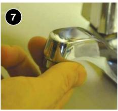
Carefully install new aerator without over tightening. Ensure rubber washers are in place and take care not to cross-thread.
