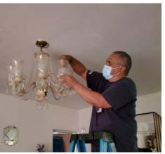
Turn off the light fixture and double check there are no safety issues such as frayed wiring or an improperly mounted fixture base. If necessary, use an appropriate ladder to safely reach the bulbs.
