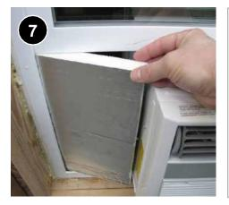
Use manufacturer-supplied side extensions and/or suitable materials to seal around the top, bottom and sides of the unit. 5.0301.1e.
