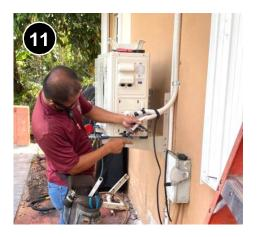
Install refrigerant lines ensuring there are no kinks, crimps, or excessive bends. Join all lines using manufacturer-approved methods. 50103.1c.
