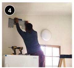
Securely fasten the mounting bracket to the wall, level, using appropriate anchors. The bracket must be installed following manufacturer specifications and in accordance with applicable building codes. 5.0108.3g.
