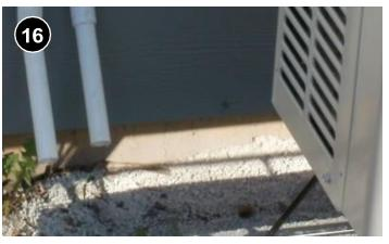
Ensure condensate can flow from the cooling unit to the exterior of the building. **5.0102.1a**.
