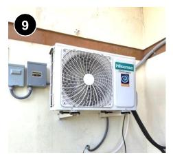
Situate the outdoor unit on a non-wicking equipment pad or stand, ensuring it is level, plumb, stable, and elevated above any potential flooding or drainage level. 5.0108.3d.
