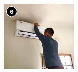
Securely mount the indoor unit according to manufacturer specifications, pushing lines through the hole you drilled, ensuring the condensate drainage is properly sloped. 5.0108.3h.
