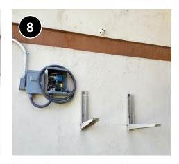
Locate the outdoor unit with manufacturer recommended clearance on all sides and to allow service access according to applicable code. 50108.3c. Also take care to ensure the total length of refrigerant piping will not exceed system manufacturer specifications. 50108.3n.
