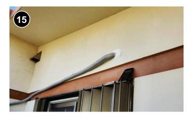
Repair all holes and damage caused by refrigerant and condensate lines passing through the building. Use appropriate materials from Appendix A that are both durable and aesthetically similar to the client's home.
