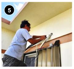
Drill hole(s) for control wires and the condensate and refrigerant lines (preferably one, but multiple if necessary).
