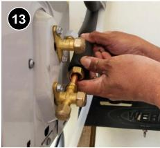
Insulate all suction lines to a minimum of R-4 with a Class II or better vapor-retarding insulation. Seal all insulation seams and joints with compatible material. All exterior insulation must be rated against UV degradation or protected from UV with another material. 5.0103.1d.
