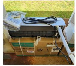
Double check the specifications of the new unit to be installed. Prior to installation, ensure refrigerant line total length will not exceed manufacturer specifications. Refer to Standard Work Specification 5.0108.3.
