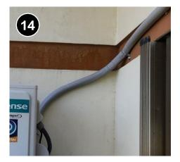
Secure and support refrigerant lines according to applicable code and in a manner that protects the lines from damage by workers or occupants. 5.0103.1e.
