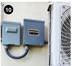
Connect wiring on the inside and outside units according to manufacturer specifications. Wires from the system must run to an electrical disconnect within sight of the outdoor unit. Best practice includes installing a surge protection device at the disconnect. All high voltage wiring must be within protective conduit and approved junction boxes. No wiring connections (high or low voltage) will occur outside of an appropriate junction box. 50108.3j.
