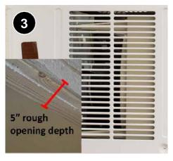
Measure the thickness from inside wall surface to the outside covering of the home. The wall thickness must not exceed the non-vented portion of the AC unit mounting assembly or unit itself (i.e., when installed, AC vents must not be blocked in any way).
