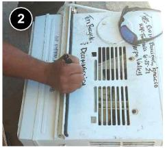
Permanently remove the old unit from the job site, taking care not to damage the wall, window, or other parts of the home. Recycle or dispose of the unit and refrigerant in accordance with local and federal law. Permanently decommission old equipment. 5.0301.1f.
