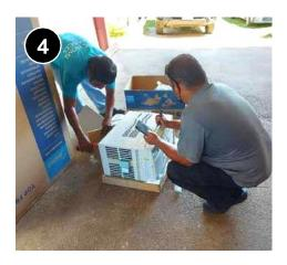
Remove the new AC until from its packaging and ensure the physical size will fit in the current hole without blocking vents. 50301.1a.
