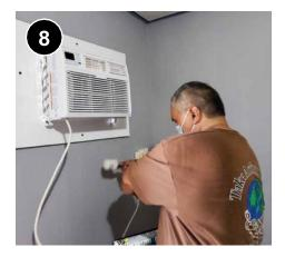
Mount the unit, leveling from left to right, keeping the unit's mounting surface flush with the inner surface of the mounting bracket, frame, or wall surface as per manufacturer instructions. Ensure the unit's condensate drain is at the lowest possible point, sloped away from the unit and the building.
