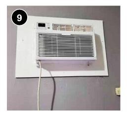
Seal the perimeter with suitable materials. Repair any excess holes in the wall opening with appropriate materials so it is aesthetically pleasing and sealed. 5.0301.1e.
