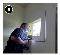
Install the mounting bracket or frame and dry-fit the unit with the help of another individual. Ensure that once the unit is mounted (according to manufacturer's instructions) it will be stable, secure, and not pose a risk to occupant safety. 5.0301.1d.
