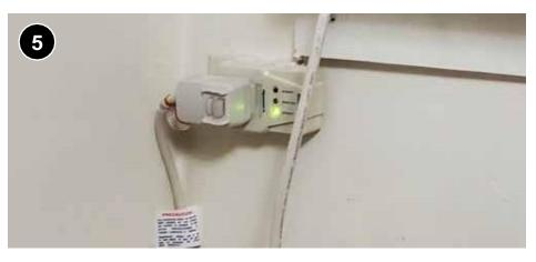
Ensure the supplied electrical cord is of sufficient length to reach the nearest outlet that meets the requirements of NFPA 70 Article 422 (Maximum breaker size for the circuit matches or exceeds the breaker marking on the appliance). It is not allowable to plug the unit into an extension cord. Therefore, if the cord does not reach, proceed with one of the following options, based on the recommendation of the auditor and available funds:
