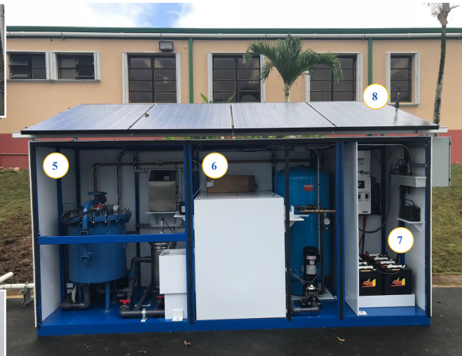
Figure 2. The main components of the pilot potable rainwater harvesting system
