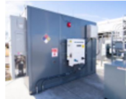
120kW – 250 kWh Lithium-ion battery
