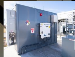
120 kW – 250 kWh Li-ion Battery
