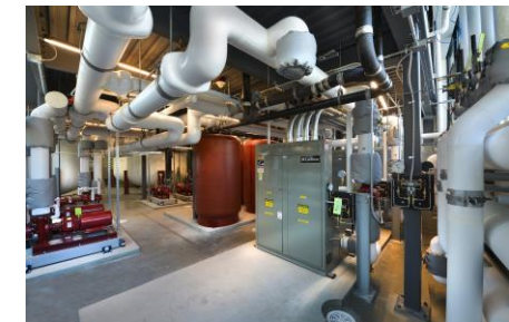
Three 8,000-gal water tanks (~187 ton-hours) five 626-gal phase-change tank (~200 to 225 ton-hours)
