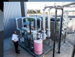
~550 ton-hours of ice storage system
