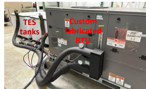
RTU modified at ORNL for charging and discharging of TES
