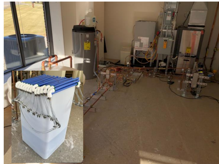
TES-integrated heat exchanger at ORNL
