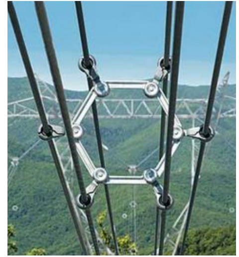
Figure 2-16. Example of bundled conductor to reduce corona effect on transmission power lines.
