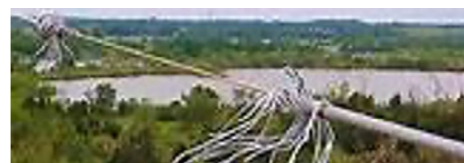
Figure A-75. Damaged conductor following the 2013 tornado.
