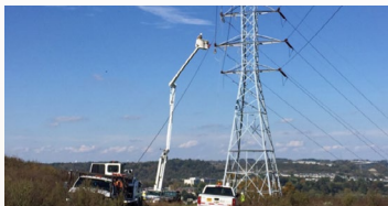
Figure A-38. Tower reconductoring.
