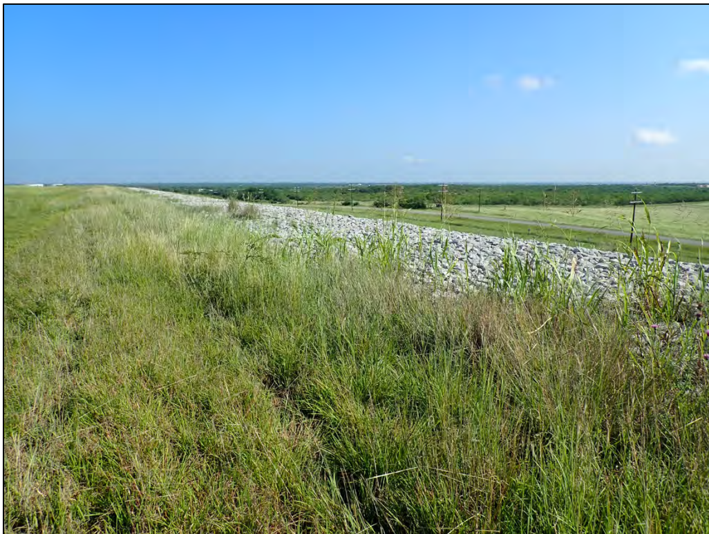
PL-8. Tall Grass Overgrown on Slide Slope Transition to Riprap
