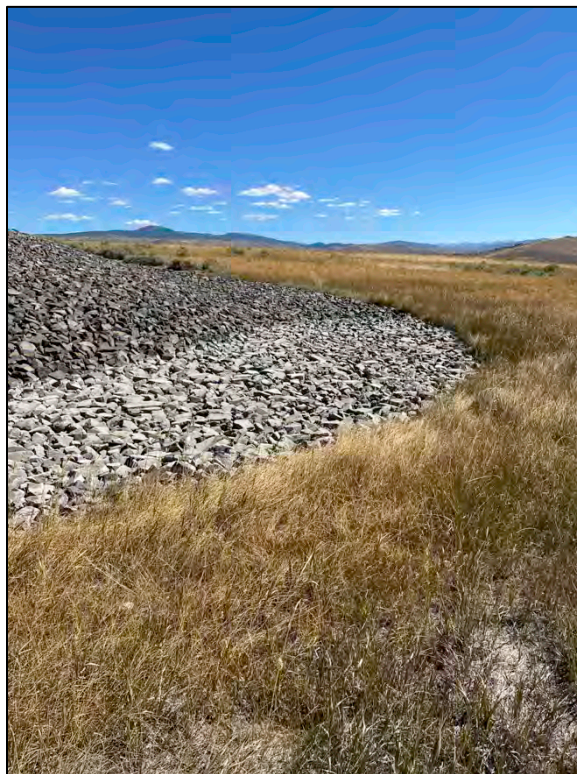
PL-6. Evidence of Water Accumulation on Southeast Toe of Disposal Cell
