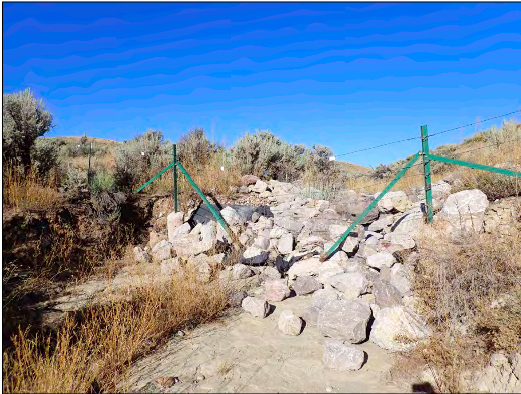
PL-7. Exposed Geofabric Below Diversion Channel No. 1
