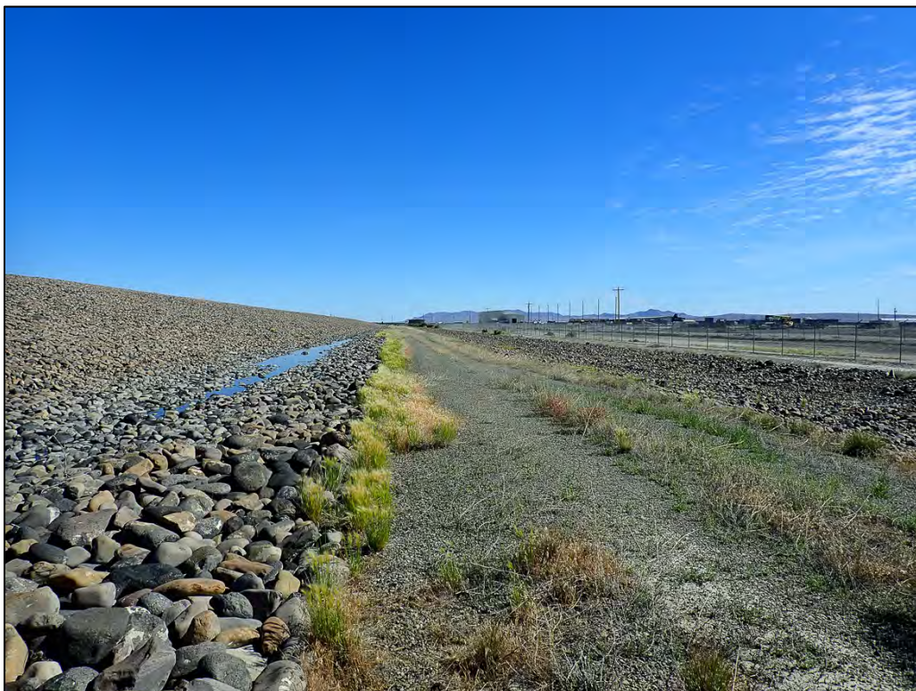
PL-9. Ponded Water in Toe Drain near Southeast Corner of Disposal Cell
