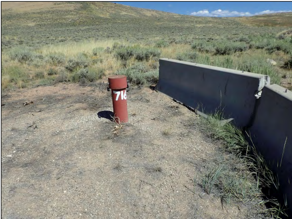
PL-4. Monitoring Well 0716 with Concrete Barriers
