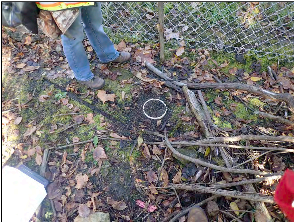
PL-6. Boundary Monument BM-2, Restored with Pea Gravel
