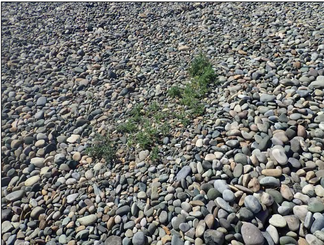
PL-4. Smaller Riprap Exposed Along Northern Ridge of Disposal Cell Top Slope
