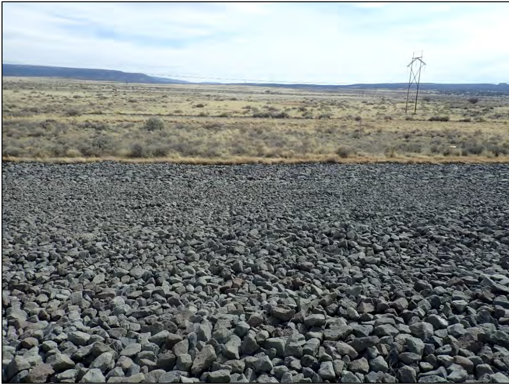
PL-9. Disposal Cell South Side Slope Toe Drain
