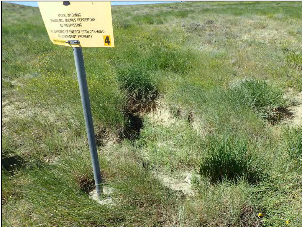
PL-3. Perimeter Sign P4 with Headcutting
