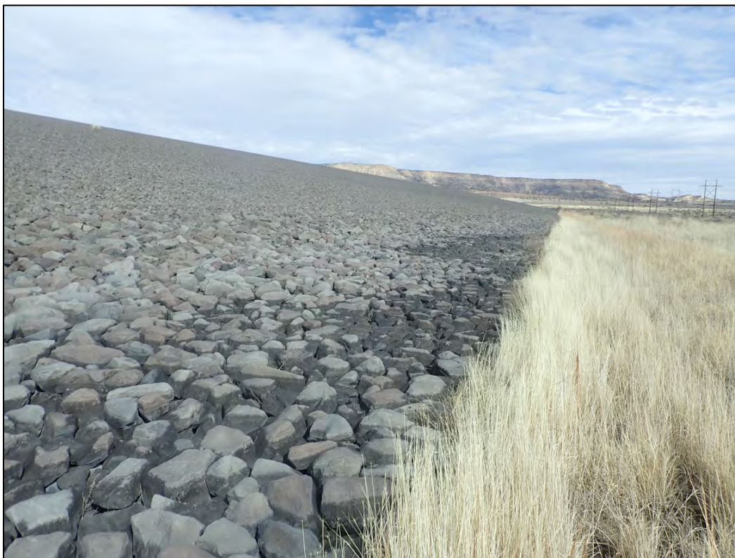
PL-8. Evidence of Ponding Water; Evaporite Forming on Riprap of Cell Apron
