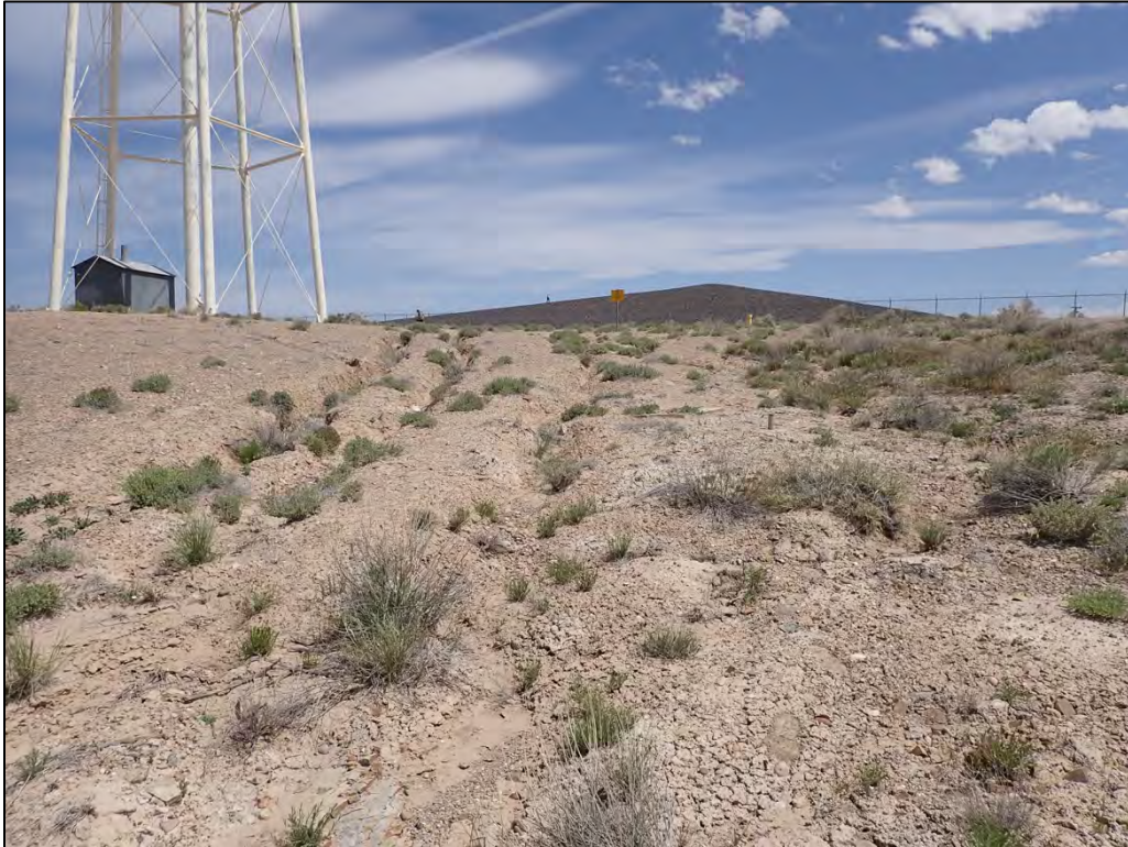
PL-7. Rills and Erosion near Water Tower
