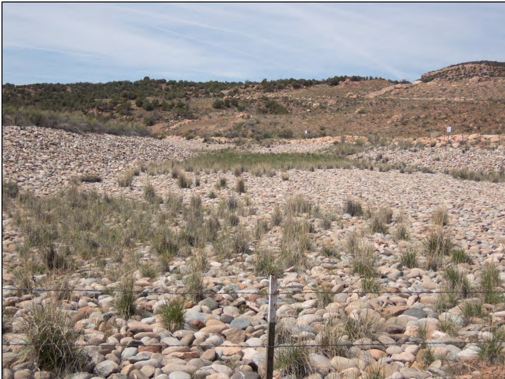
PL-8. Interceptor Trench on Northern Side of Disposal Site
