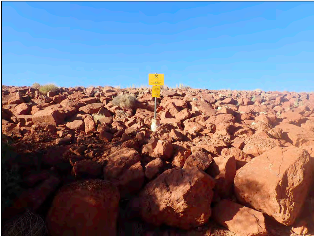
PL-3. Perimeter Sign P7 with Exposed Base
