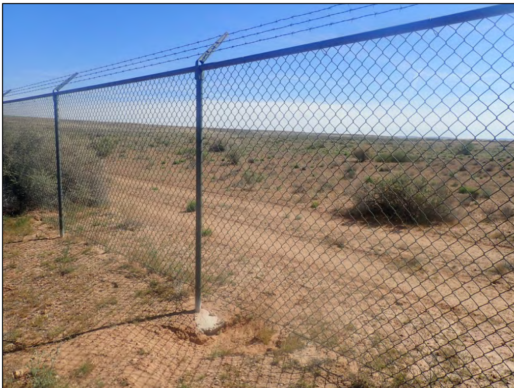
PL-2. Gap Created by Animals Under Fence Between Perimeter Signs P21 and P22
