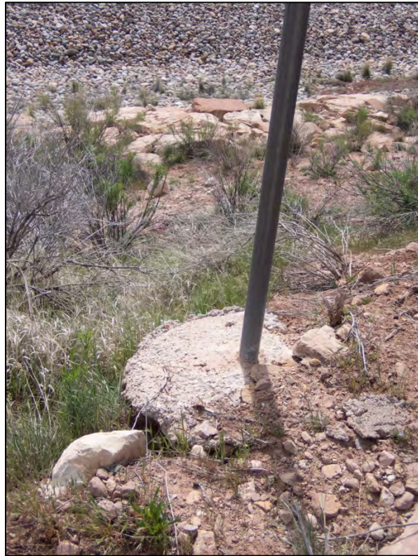
PL-3. Erosion Around Concrete Base of Perimeter Sign P22
