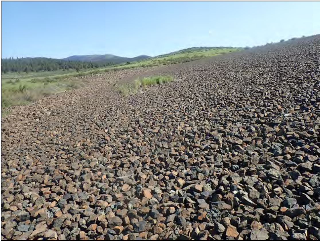
PL-11. Grass Patch on Riprap Between Water Flux Meters WFM2 and WFM3
