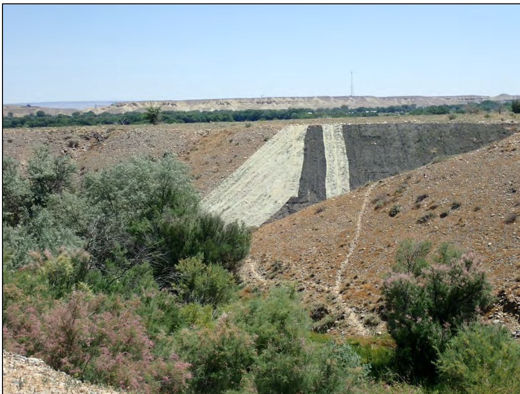
PL-7. Repaired Erosion Control Fabric
