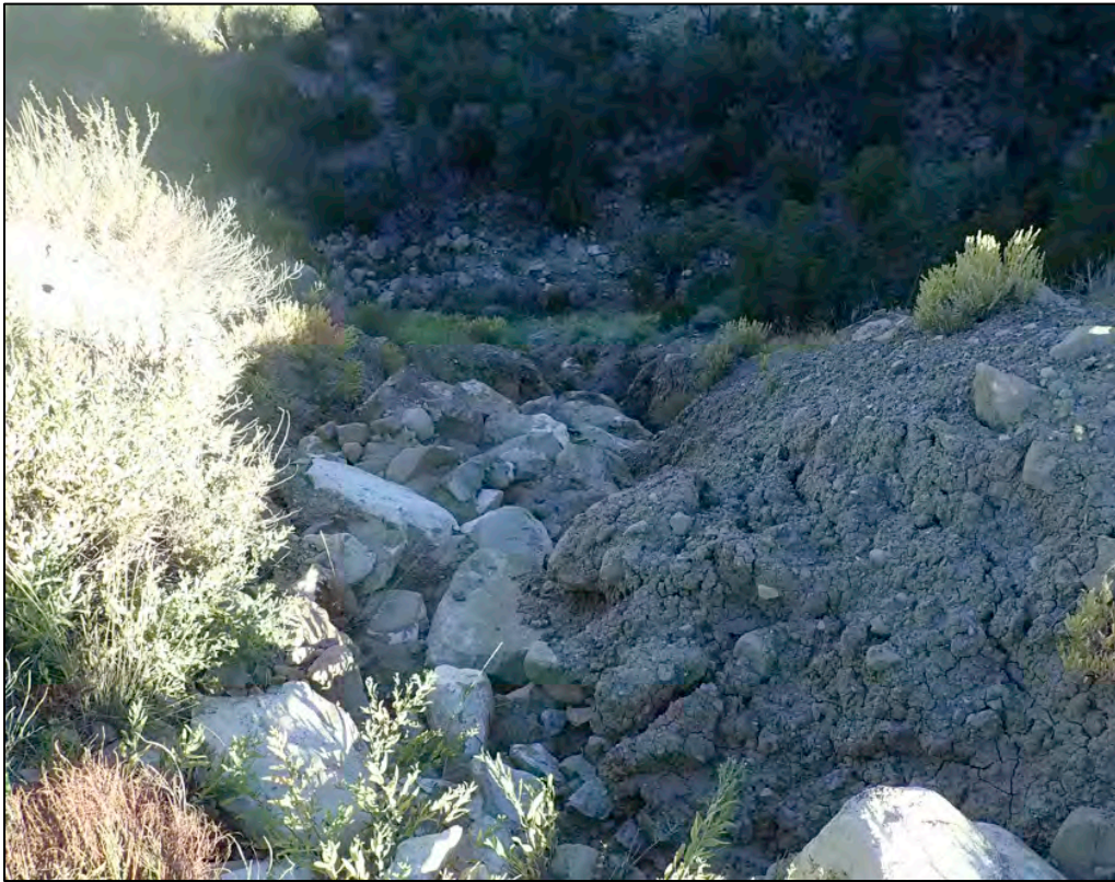
PL-9. Gully at Toe of Interceptor Trench
