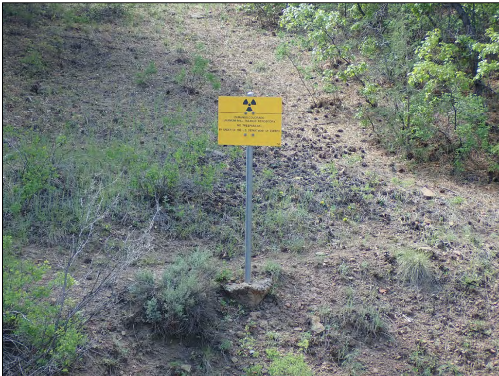
PL-2. Undercutting Around Base of Perimeter Sign P56
