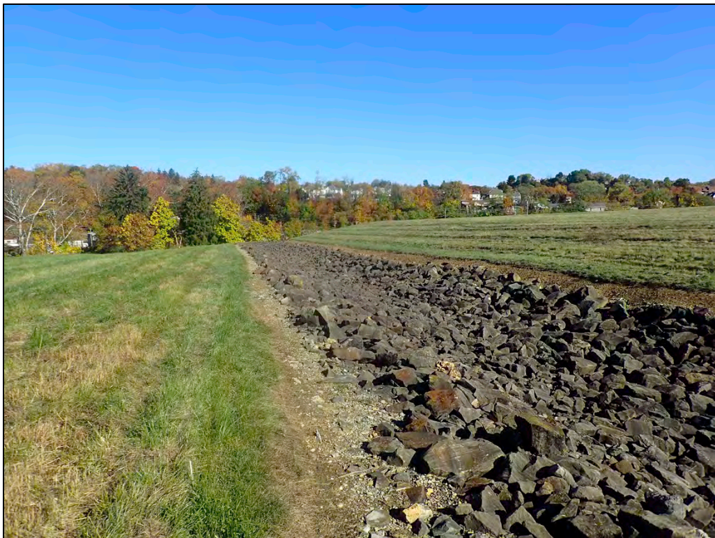
PL-10. Looking North Down Riprap-Armored Diversion Channel
