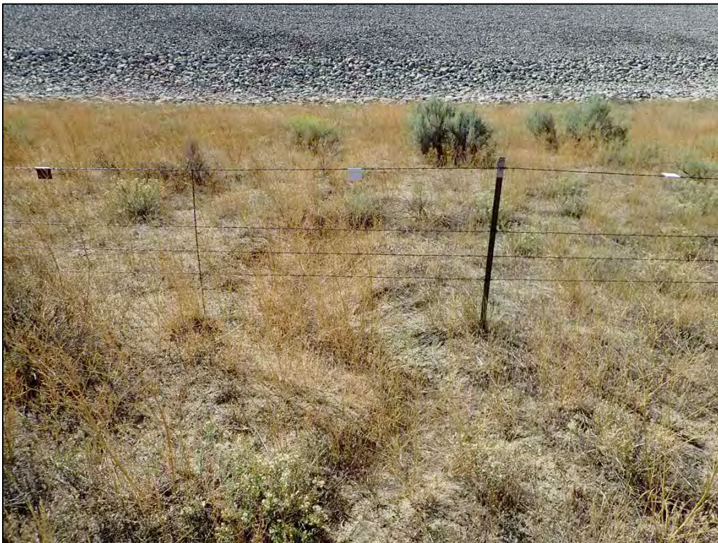
PL-10. Minor Rilling Under Fence
