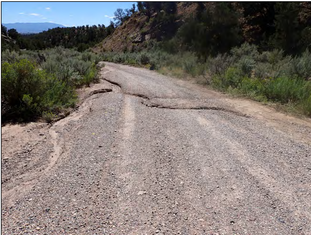
PL-2. Rutting and Erosion Along Access Road
