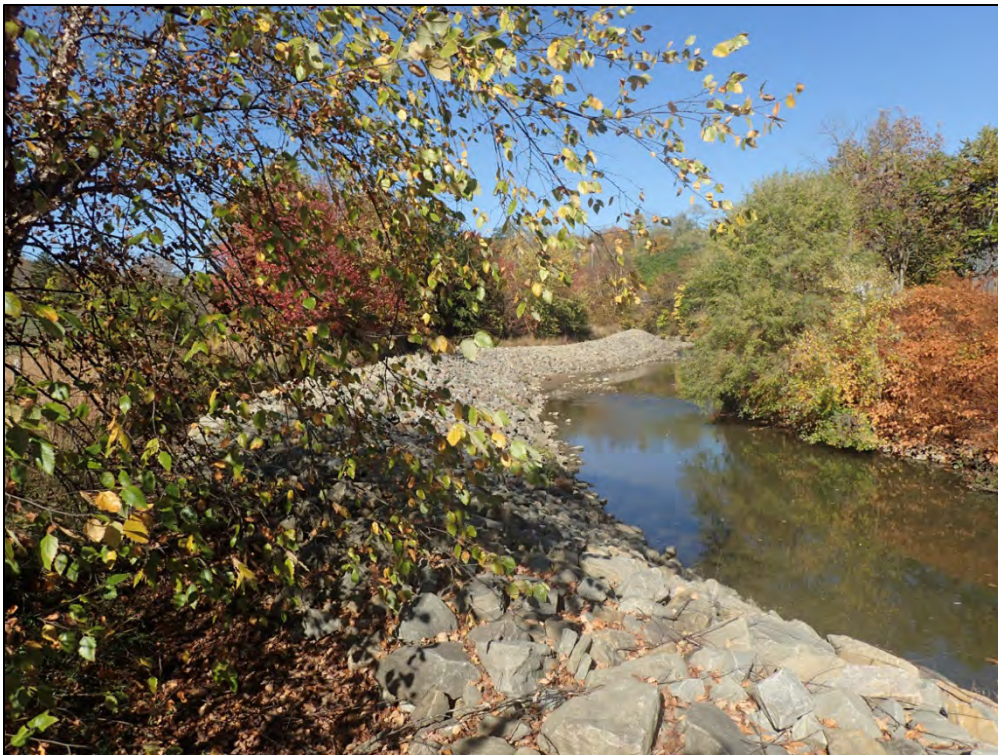
PL-12. Riprap-Armored Streambank
