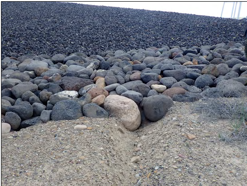
PL-6. Rill Running into Toe Drain near North Corner of Disposal Cell
