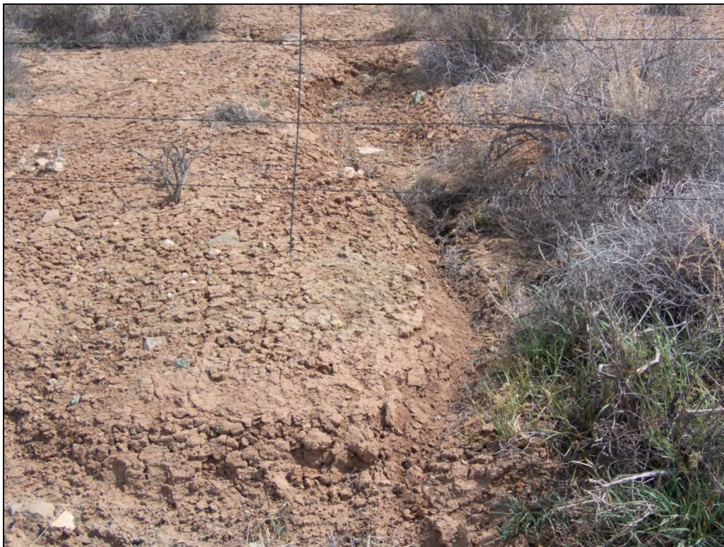
PL-2. Gully Forming Under Fence Line Along County Road T11
