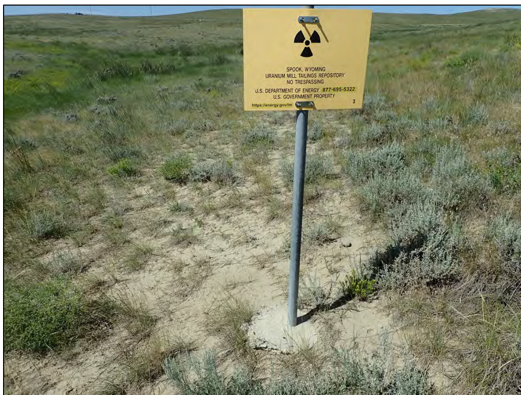
PL-2. Perimeter Sign P3 with Headcutting
