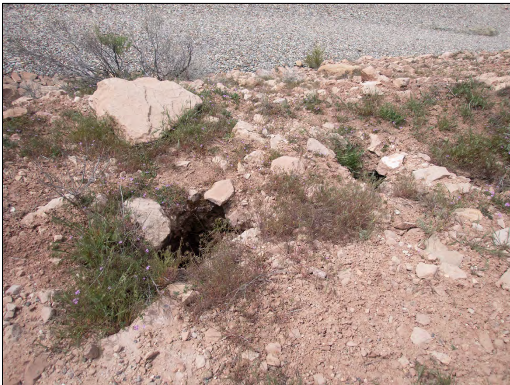
PL-12. Erosional Channeling Along North Cliff Above Disposal Cell
