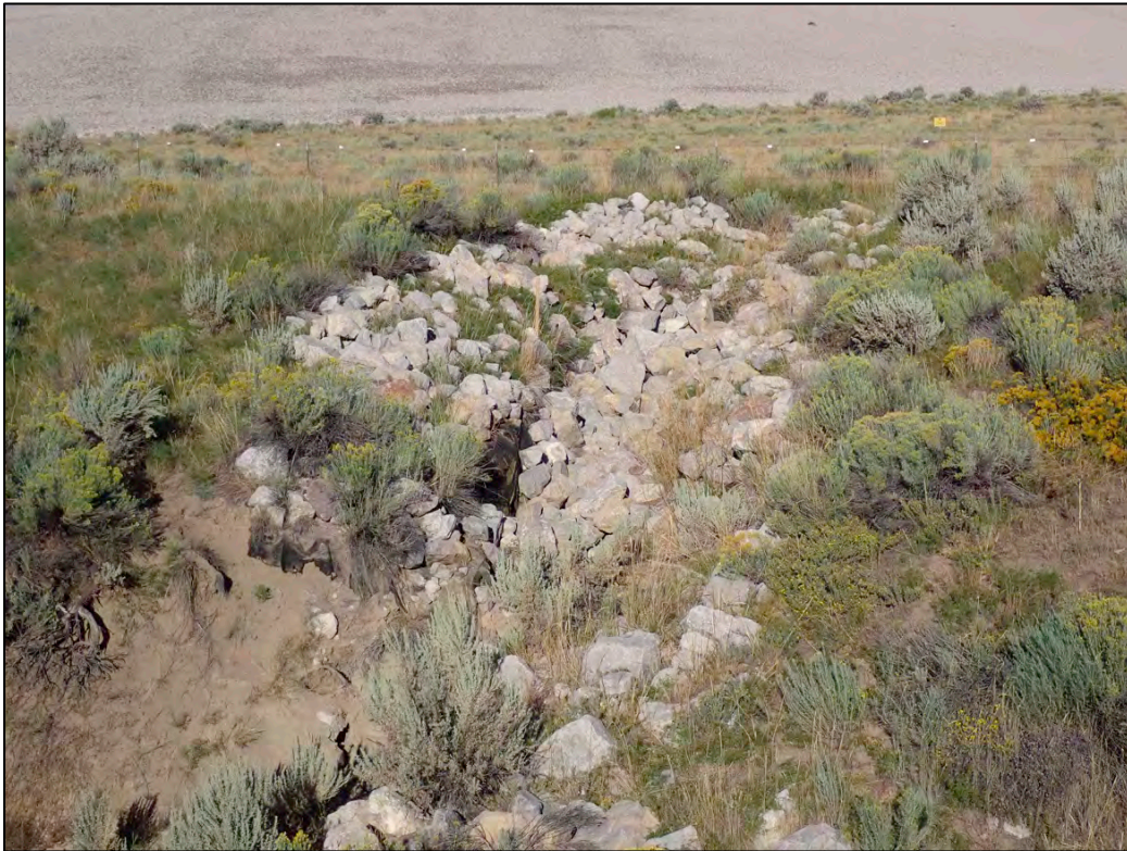
PL-9. Exposed Geofabric in Swale No. 2
