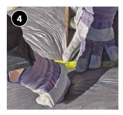
Cut batt to length for cavity and trim the width if needed to ensure a proper fit.
