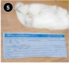
When complete, post a dated insulation certificate/receipt signed by the installer with the required information (e.g., insulation type, area insulated, thickness, etc.).
