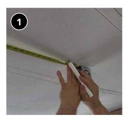
Prior to drilling evenly spaced access holes, confirm the structural integrity of the roof assembly and ensure no roof leaks exist.
