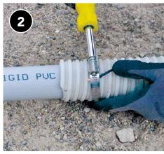
Clamp a piece of copper wire to a metal connector to discharge static electricity build up.
