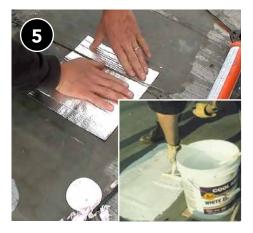
Install a flexible adhesive roof patch over the first patch. When complete, apply a final coat of elastomeric paint over the affected area.
