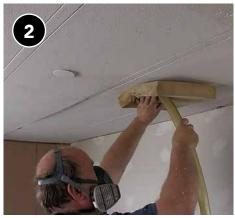
Blow loose fill fiberglass insulation to the correct density while ensuring complete coverage.
