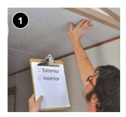
Verify the integrity of the ceiling to ensure it can support the weight of additional insulation.
