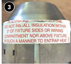
Replace non-insulation contact rated can lights with insulation contact-rated cans.
