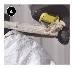
Clean old butyl tape or putty from J channel and store J channel somewhere safe until it can be reinstalled.
