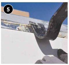
Remove staples holding down edge of roof.
