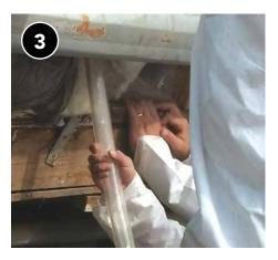
Fill cavity with blown fiberglass insulation; carefully maneuver the fill tube past the belt rail and around the electrical boxing/wiring.
