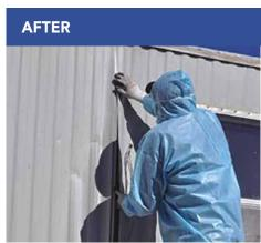
When properly insulated, siding should not bulge or be dented as a result of the installation. Document the location of any pre-existing dents and point them out to the building owner prior to starting a project.
