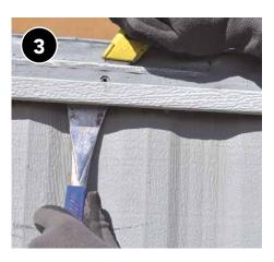
Unfasten and remove J channel from edge of roof.
