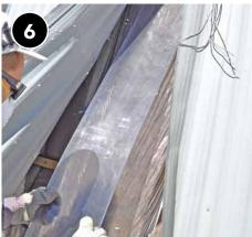
Insert batt into cavity, sliding under top belt rail to top of cavity, and pull the stuffing tool back out to allow batt to fill in space.
