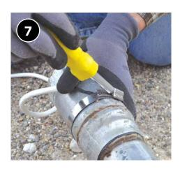
Ground fill hose to reduce chance of electrical buildup.
