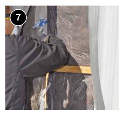
Gently tug batt into place, tuck remaining batt under lower belt rail, and fit down to bottom of cavity with minimal compression.
