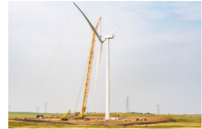
Erect Wind Turbines
