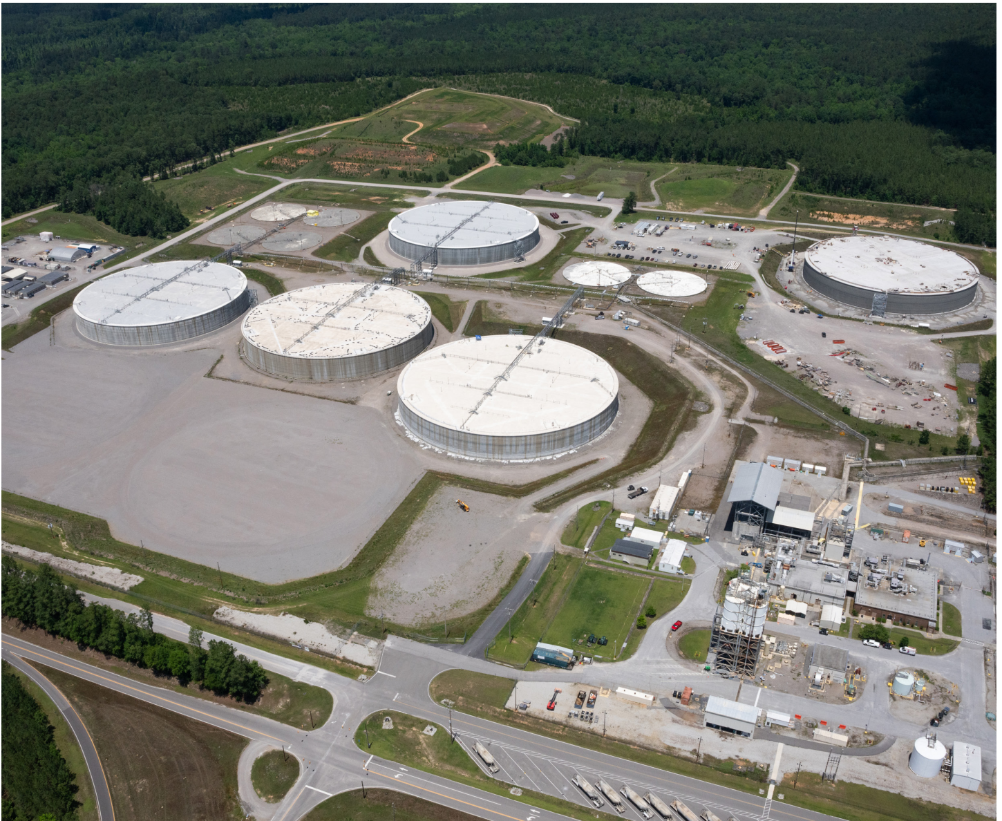
Saltstone Disposal Units are permanent disposal units at the Savannah River Site. The smaller SDUs can be seen alongside the larger, mega-volume SDUs.
