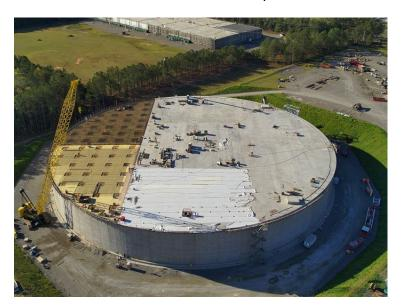
All major concrete placements have been completed on Saltstone Disposal Unit 10, the latest mega-size disposal unit being built at the Savannah River Site, bringing the U.S. Department of Energy Office of Environmental Management and contractor Savannah River Mission Completion a step closer to achieving the liquid waste mission. This aerial view shows the final roof section being installed on the unit.
