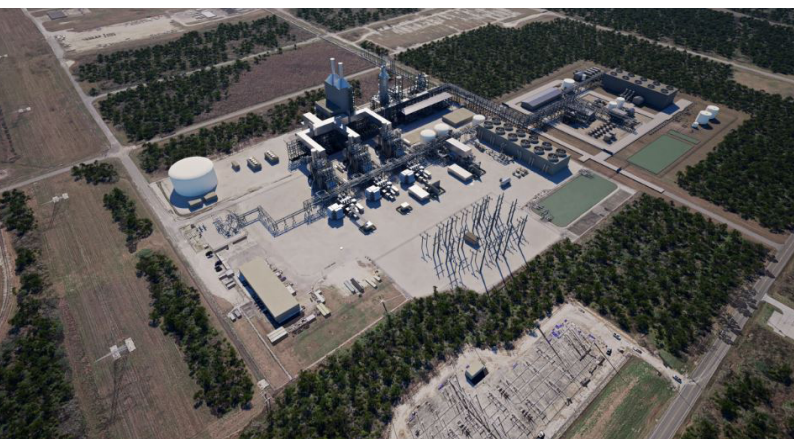
The Baytown Carbon Capture Project plans to use Shell's CANSOLV point-source technology to capture up to 2 million metric tons of CO 2 annually—equivalent to the annual emissions of nearly 450,000 gasoline-powered cars.
