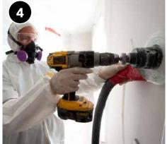
Drill insulation access holes as needed to ensure complete coverage of all uninsulated wall cavities.
