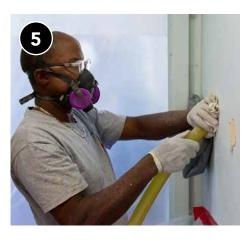
Fill cavities completely and to the proper density.
