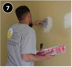
Patch insulation access holes or use a chair rail molding to cover the holes.
