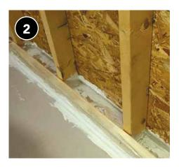
Ensure balloon-framed walls are blocked at top and bottom to prevent insulation from unintentionally blowing into the attic or basement.
