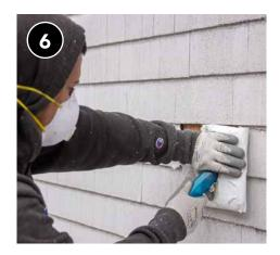
Using an injection fill tube, insulate all cavities to the proper density.
