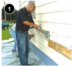
Protect work area from debris and dirt before removing siding.
