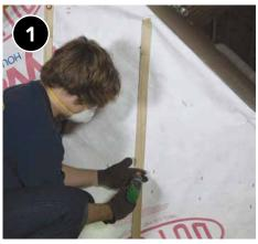
Securely install backing material over entire attic wall to create an enclosed cavity. Use wood strips along the studs and edges of the framing to hold the material in place, withstand air pressure, and prevent insulation from spilling out.
