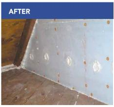
Once insulated, this attic wall provides a continuous, contiguous, safe, and compliant thermal boundary that prevents air movement. When using rigid foam insulation as the backer material, ensure the material meets fire safety requirements of the authority having jurisdiction.
