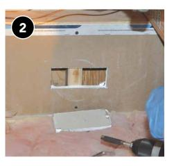
Cut holes in rigid backing material or cut small slits in house wrap material to allow access to each cavity.
