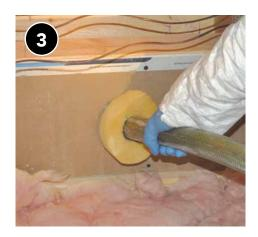
Blow insulation into cavities to meet dense-pack standards.
