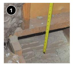
After clearing away debris, measure gap below knee wall in line with pressure boundary.
