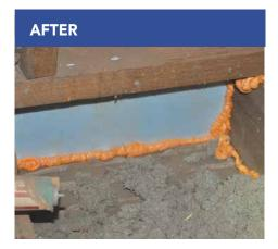
Air sealing each and every open joist cavity below the knee wall prevents air movement between the unconditioned attic and the conditioned floor.
