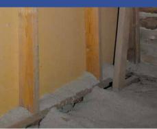
Knee walls often define the thermal and pressure boundary and the open joist cavity below requires careful air sealing.
