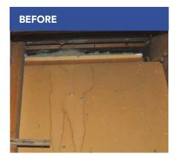
Knee walls often define the thermal and pressure boundary. Above the knee wall is often an open roof rafter cavity, which may need blocking or the knee wall could be missing a top plate.
