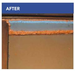
Air sealing the top of a knee wall continues the pressure boundary while supporting additional insulation from the knee wall or roof rafter above.
