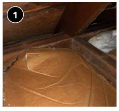
After clearing away debris, measure gap above knee wall in line with pressure boundary.
