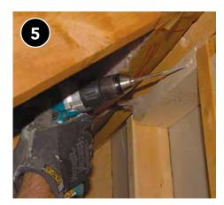
If a top plate is required, secure wood in place with mechanical fasteners.
