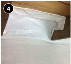
An alternative method to steps 1–3 is to bring rigid foam or house wrap material up to the roof decking to block the opening and create an air seal when the edges of the material are sealed to the framing.
