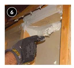
Seal blocking with mastic, caulk, or one-part foam to maintain the pressure boundary and prevent air movement within the cavity.
