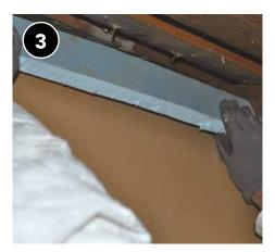
Securely fit infill or blocking material in place and seal around the edges.
