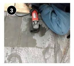
Prepare the area around the hole before installing a metal patch.
