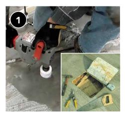
Cut access holes (rectangular or round holes) large enough to fit a fill tube in each cavity.
