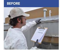
Confirm the structural integrity of the roof assembly and verify no active roof leaks exist prior to installation.
