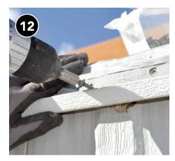
Reattach J channel, lapping over edge of roof. Repeat entire process for other side, if necessary.
