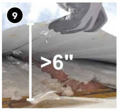
Work down the edge of the roof until entire cavity is full.
