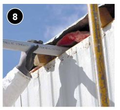
Insert blower hose as far as possible into cavity and retract slowly while filling space between trusses.
