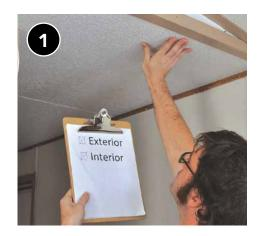
Verify the integrity of the ceiling to ensure the ceiling can support the weight of additional insulation.
