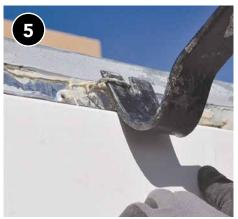
Remove staples holding down edge of roof.
