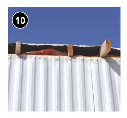
Remove blocks and reattach edge of roofing over exterior sidewall paneling.
