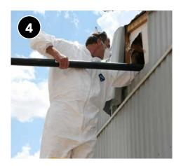
Insert the insulation fill tube as far as possible, moving the tube side to side while slowly retracting it to ensure adequate insulation coverage. If a marriage wall is present, use this technique on each side of the wall.
