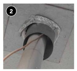
Dam around high-temperature flues (note: flue in image is in need of work).
