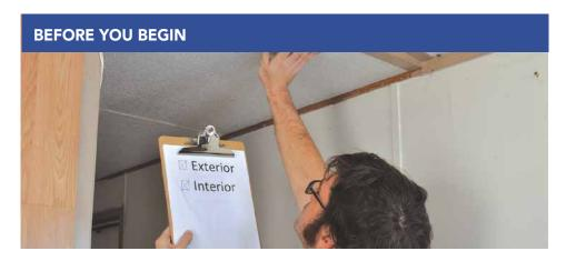
Make any repairs and preparation as noted from assessment, as well as fixing any new issues that could cause the ceiling to be compromised because of the additional weight of insulation.
