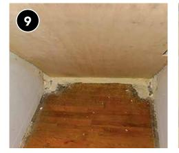
Cover insulation with an approved thermal barrier material for fire safety and to seal off insulation from conditioned space in home.
