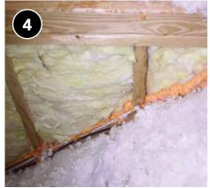
Cut batts to size for each individual cavity, ensuring no gaps remain, locating insulation vapor retarder toward conditioned space.
