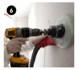
If walls are enclosed from attic side, drill holes in stairway walls defining the thermal boundary.
