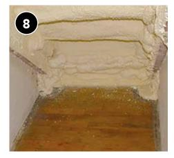
If the stairs have no backing material (e.g., drywall, plaster, etc.) towards the house or conditioned space; insulate with material specified by the work order.
