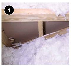
If walls defining the thermal boundary are accessible from the attic side, choose between batt or blown-in insulation.
