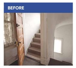
Attic stairways can offer a unique set of insulation challenges. Clearly define where the thermal and pressure boundary are going to be located before starting insulation.
