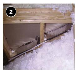
Seal off open cavities along the line of the thermal/pressure boundary.
