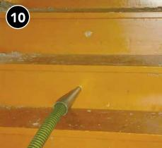
If backside of stairs already have backing material, blow insulation into cavity behind stairs.
