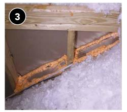
Air seal around blocking material.
