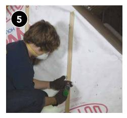
For batt insulation, cover installed batts with backing. For blown-in, attach netting to framing members, cut holes in netting, and blow insulation to an installed density of 3.5 pounds per cubic foot.
