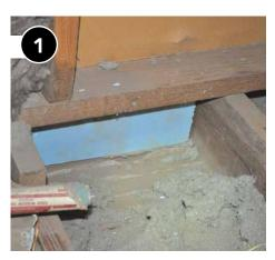
Ensure that floor cavities and chases are blocked securely at both ends with all edges of the blocking sealed.
