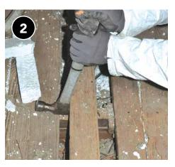
If boards can be loosened, pry up as few boards as possible to access all cavities. If flooring is in solid sheets, access holes may need to be drilled.
