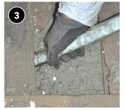
Fill entire cavity with insulation to prescribed density. Reinstall any boards removed and close any access holes when complete.
