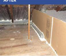
An insulated attic floor provides a continuous, contiguous, safe, and compliant thermal boundary that reduces air movement.
