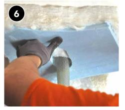
Blow insulation to completely fill cavities to prescribed density.
