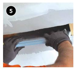
Blocking still needs to be put into place if open cavities extend into conditioned space (e.g., cavity below a knee wall in an outer ceiling joist attic space).
