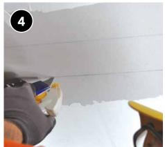
Occasionally, a homeowner may not want the attic floor to be disturbed. The cavities can also be accessed from below through the ceiling, particularly in garages.
