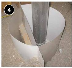
Ensure that insulation does not get into dammed-off areas, such as around chimneys and flues and inside soffit baffles.
