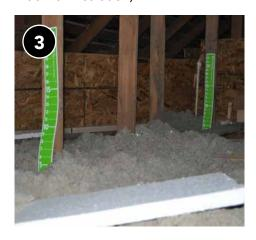
While installing, regularly check depth of insulation for even coverage and to meet required depth.
