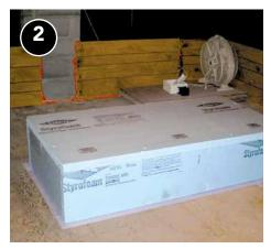
Insulate top and sides of dam cover, to appropriate R-value. Use materials that meet the requirements of the applicable fire safety code (e.g., thermal or ignition barriers).
