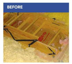
Pull-down stairs can be a weak point in thermal/pressure boundaries, and they can also allow insulation to fall into the home if not properly dammed.
