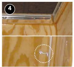
Air seal with closed cell foam tape or weatherstripping. Install latches as needed to ensure the access door closes tight to the weatherstripping.
