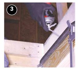
Air seal gaps in framing and edges of trim as needed.
