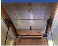
Attic pull-down stairs are safely and durably sealed and insulated to prevent air movement and reduce heat transfer.
