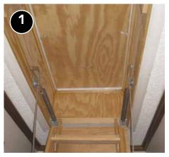
Build cover above and around pull-down stair, taller than final insulation height.
